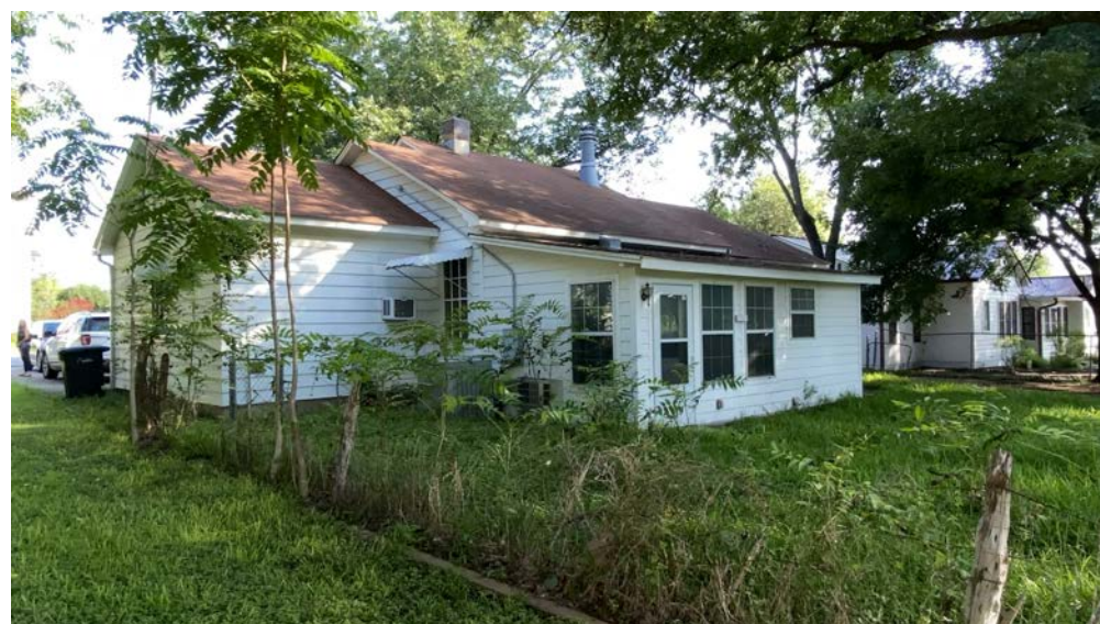
REAR OF EXISTING BUILDING SHOWING GARAGE AND REAR ADDITION
