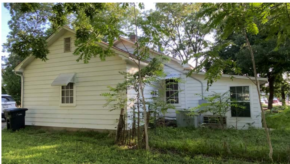
SIDE OF EXISTING GARAGE
