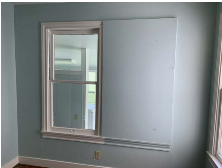
WINDOWS THAT HAVE BEEN COVERED OVER/ENCAPSULATED BY REAR ADDITION
