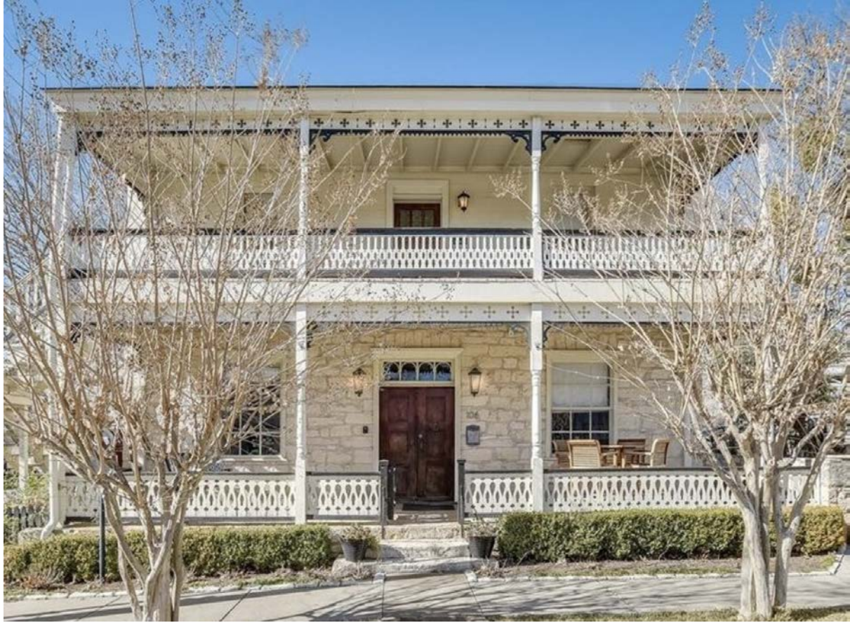
Existing condition at 106 South Lincoln - Not compliant with safety & building code
