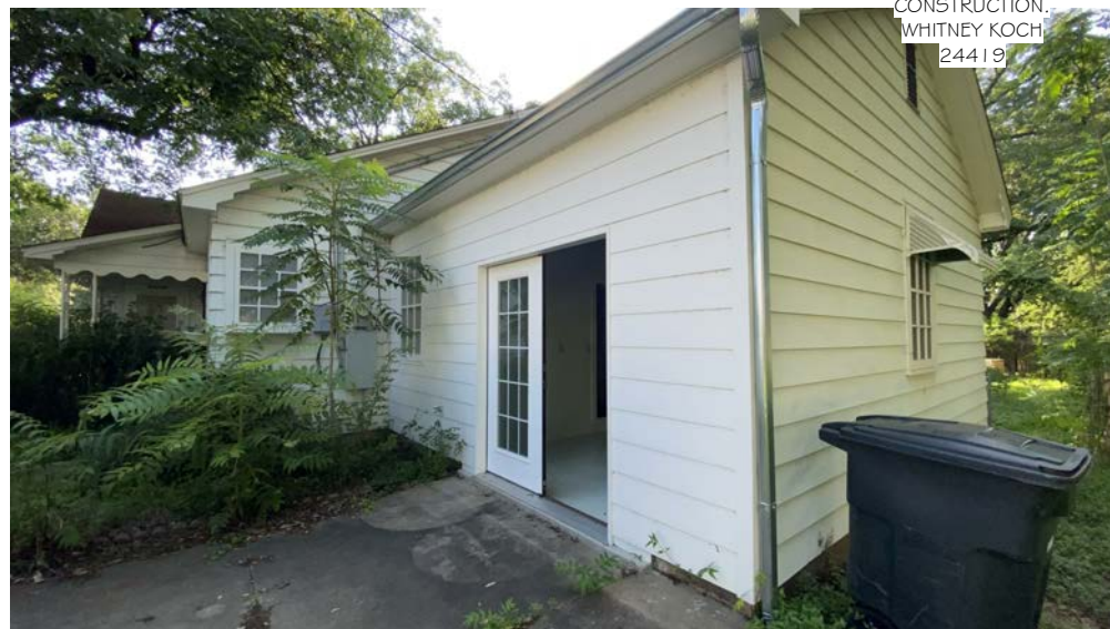
FRONT OF GARAGE WITH CEMENT BOARD SIDE AT FRONT AND SIDE (DOES NOT MATCH RESIDENCE)
