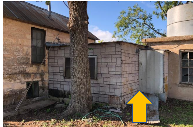
Remove wood framed infill – Protect tree.
