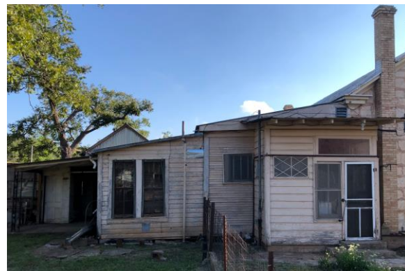
South view of wood framed lean to be removed.
