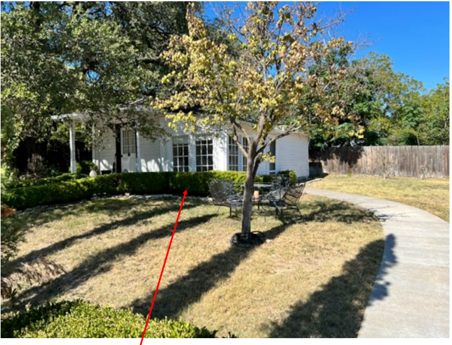
Historic aged ADU with non-historic lean-to addition (to be removed)
