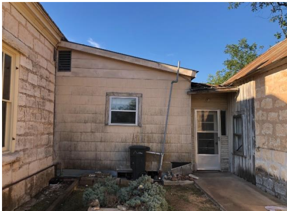
Close up view of lean to addition to be removed
