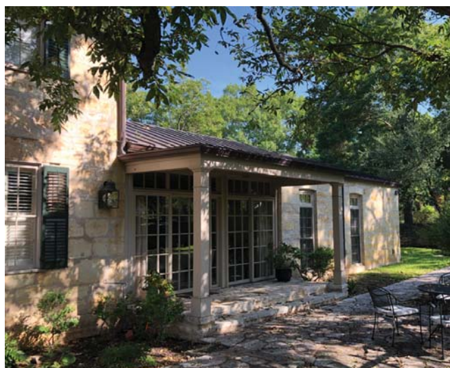
Existing SE view of 2012 Additon
