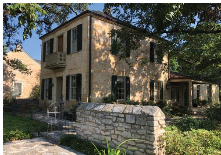
Existing Southeast view
