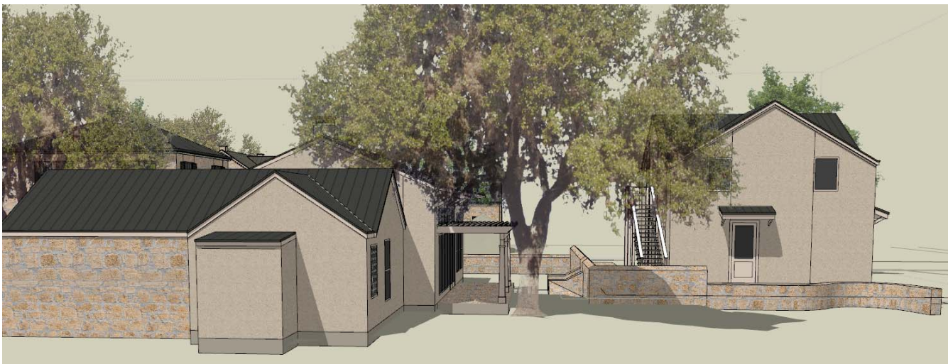
Northeast rear yard View
