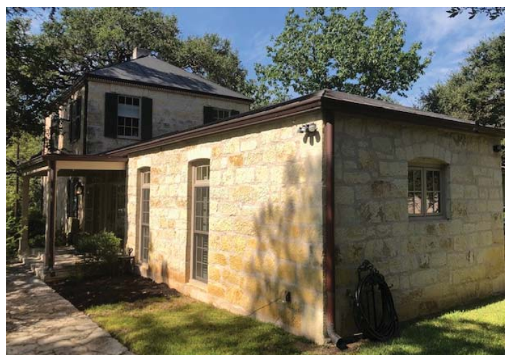
Existing NE view of 2012 Additon
