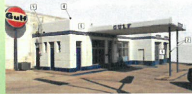
Figure 10-18. Constructed c. 1940; located at 301 North Locust Street, Denton, Denton County.
