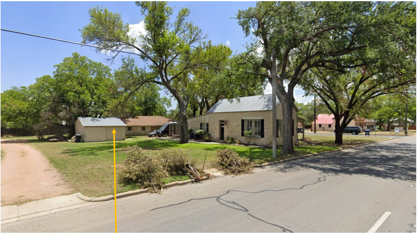
Ca 1940's garage behind 1880's stone house
