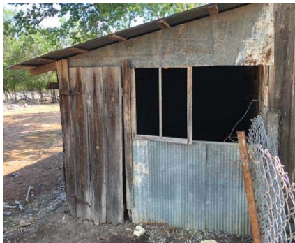
South close-up of lean-to
