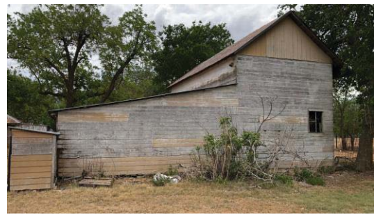
North Elevation of barn
