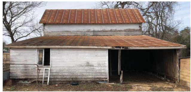
East elevation of barn
