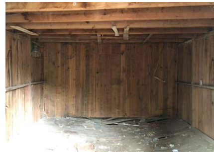
Interior view of barn – collapse floor.
