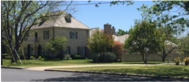
Figure 3 Example of polymer composite shingles at 707 West Creek Street
