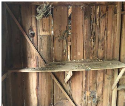
Close up view of barn siding w/ collapsed floor
