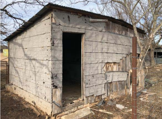
Southeast view of the storage room.
