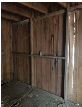
Close up view of barn siding w/ collapsed floor
