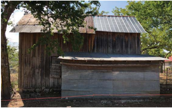
West elevation of Barn
