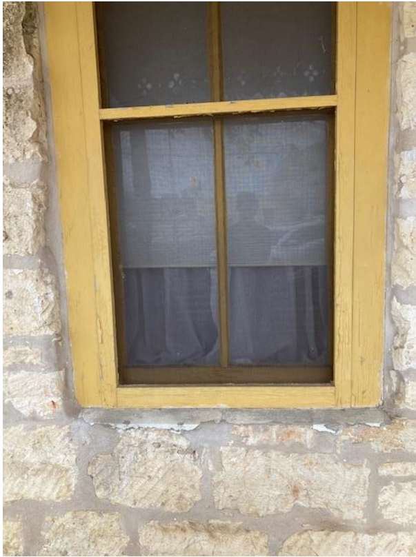
Figure 4 Rough edges caused by 1920s window enlargements
