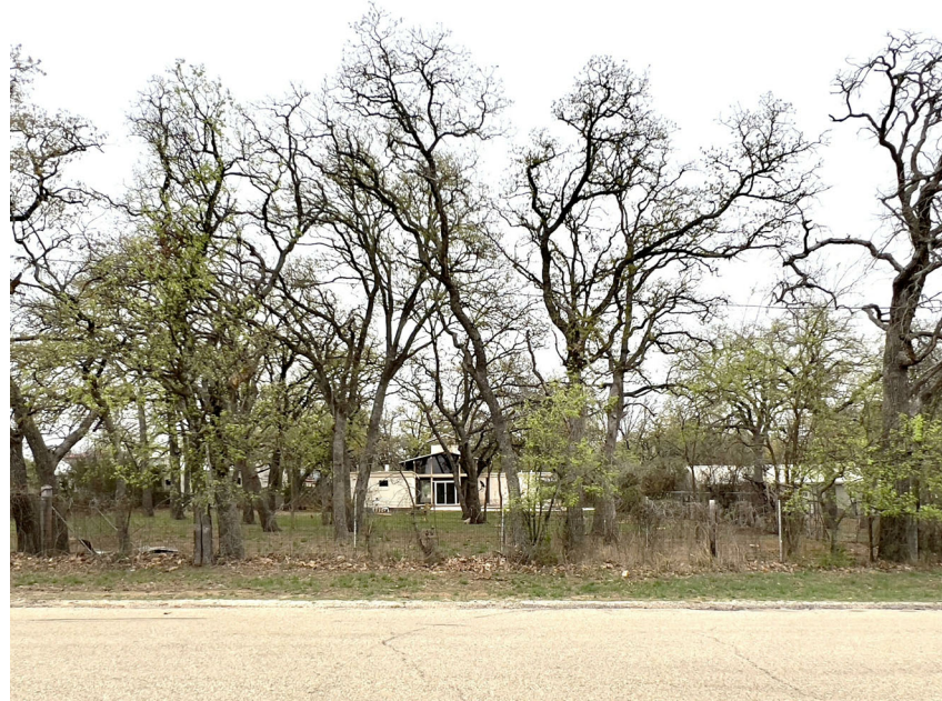
EXISTING RESIDENCE, IMAGE ALONG CATHOLIC CEMETARY ROAD
