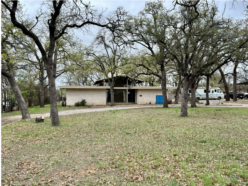
EXISTING RESIDENCE, IMAGE ALONG WOODCREST STREET
