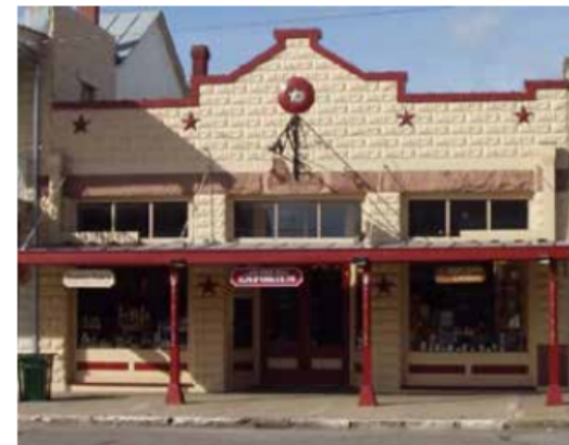
Figure 3-37. Example of an appropriate canopy on a historic building at 121 E. Main Street. Note how the canopy is mounted so that it does not obscure the transom windows above. Also note the metal tie rods anchored into the façade. Source: HHM 2003 Historic Resources Survey.
