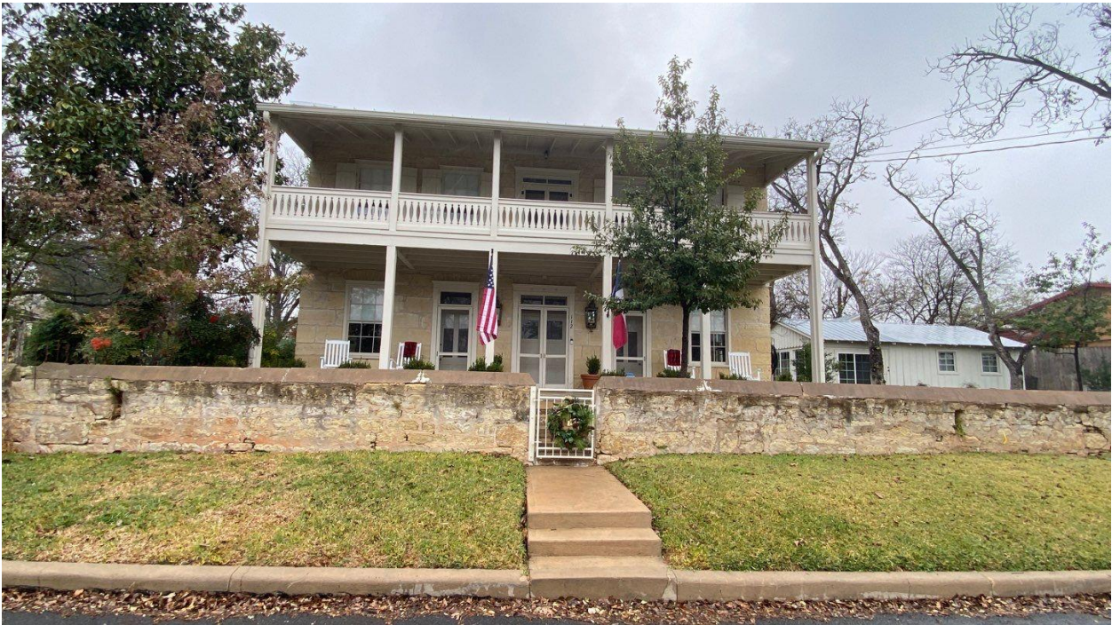
Views of elevation and fencing facing the front of the property
