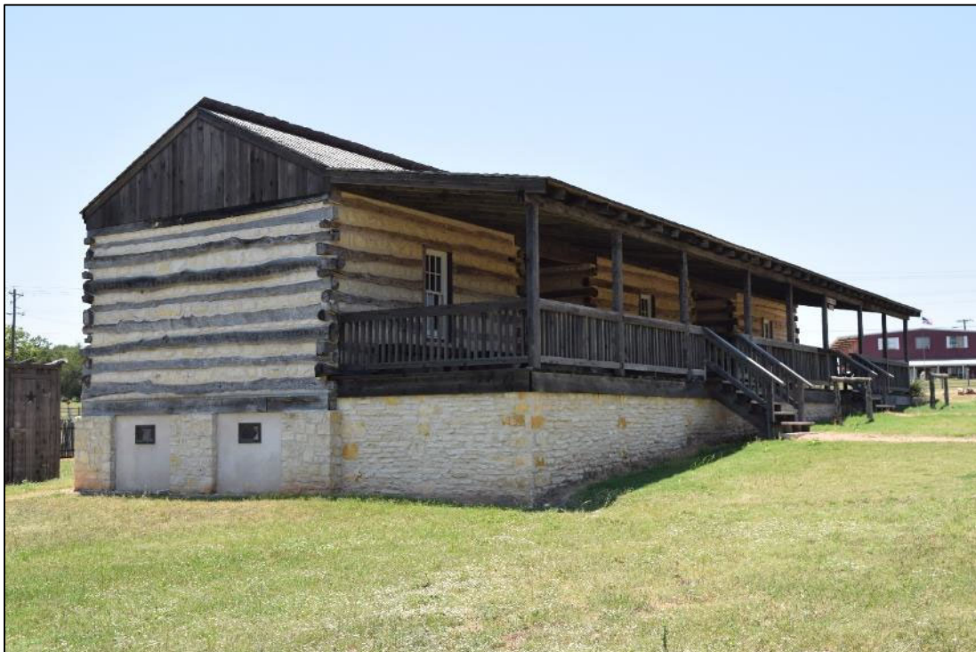
Figure B-40. Building R., the Enlisted Men's Barracks, facing east.
