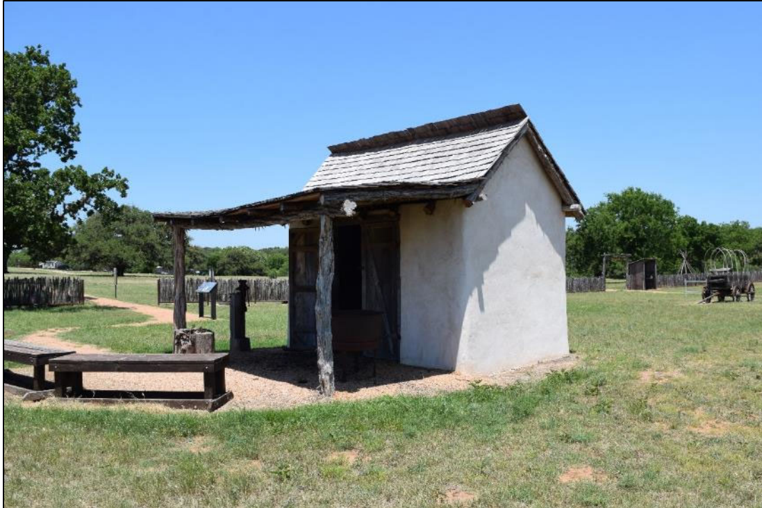
Figure B-43. Building V, the Blacksmith Shop, facing south.
