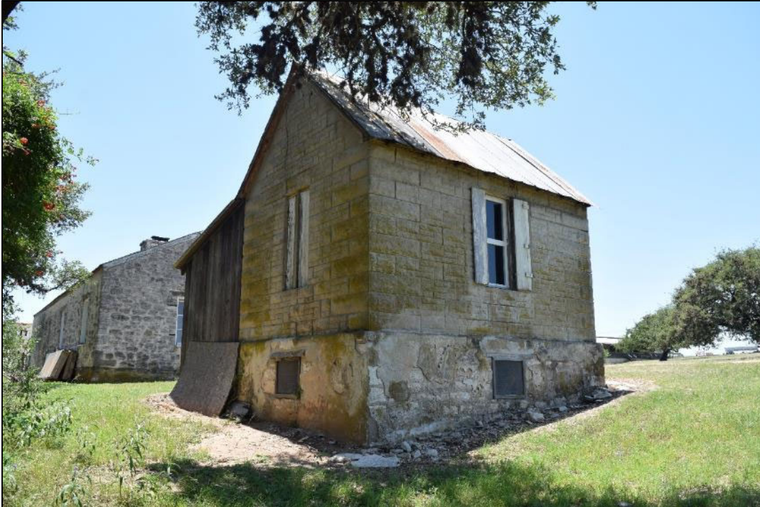
Figure B-35. Wash House (Braeutigam Shed), facing southwest.
