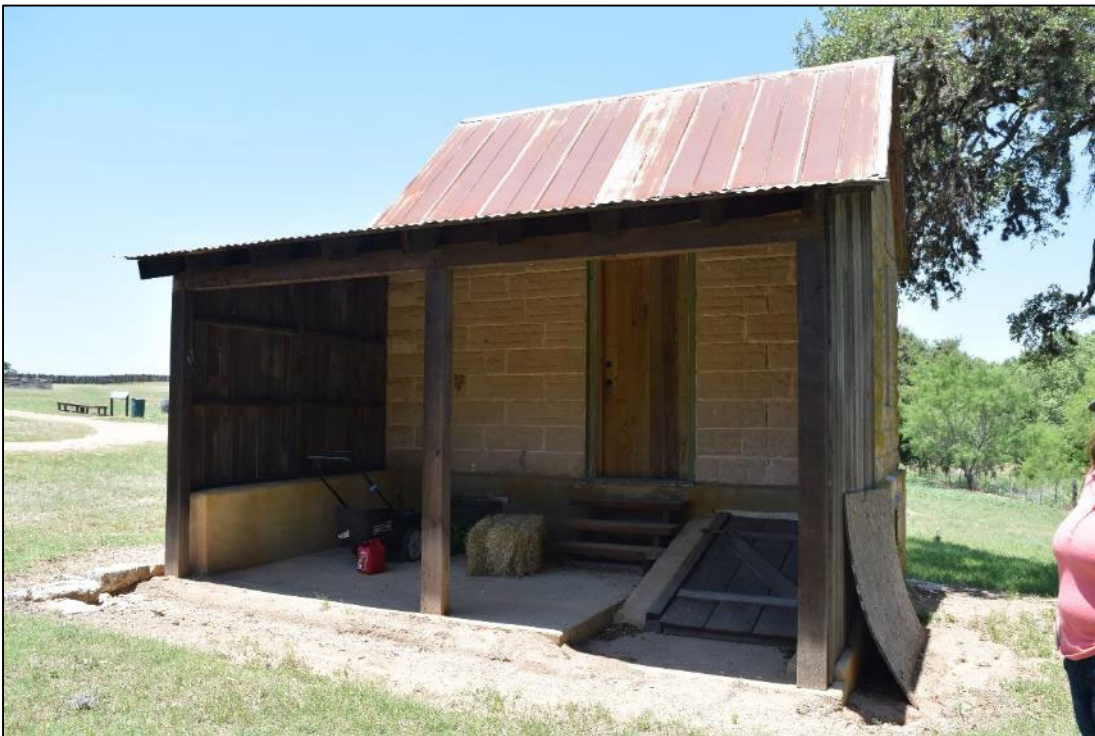
Figure B-36. Wash House (Braeutigam Shed), facing north.
