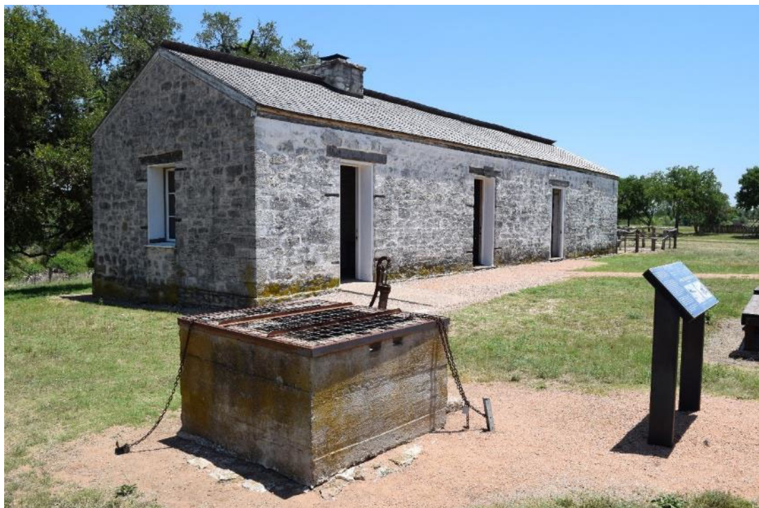
Figure B-30. Building N, the Guard House, with Braeutigam Well #1 in foreground, facing south.
