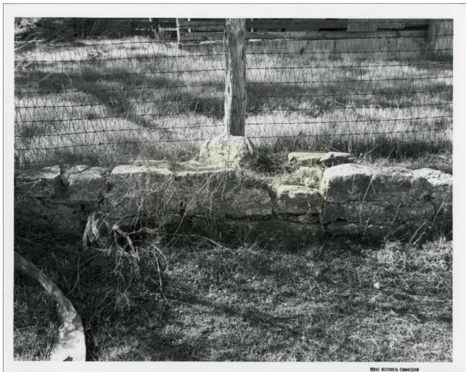
Figure 5. Detail of stone foundations of ruins, specific building and view not noted (NRHP 1979).
