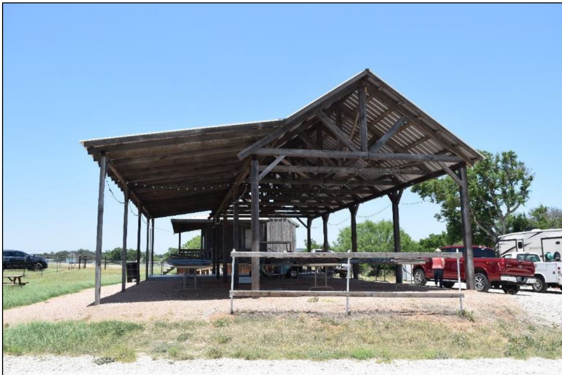
Figure B-48. Wagon Barn, facing north.
