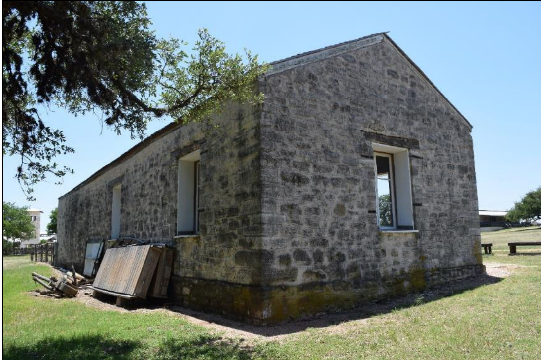
Figure B-31. Building N, the Guard House, facing southwest.
