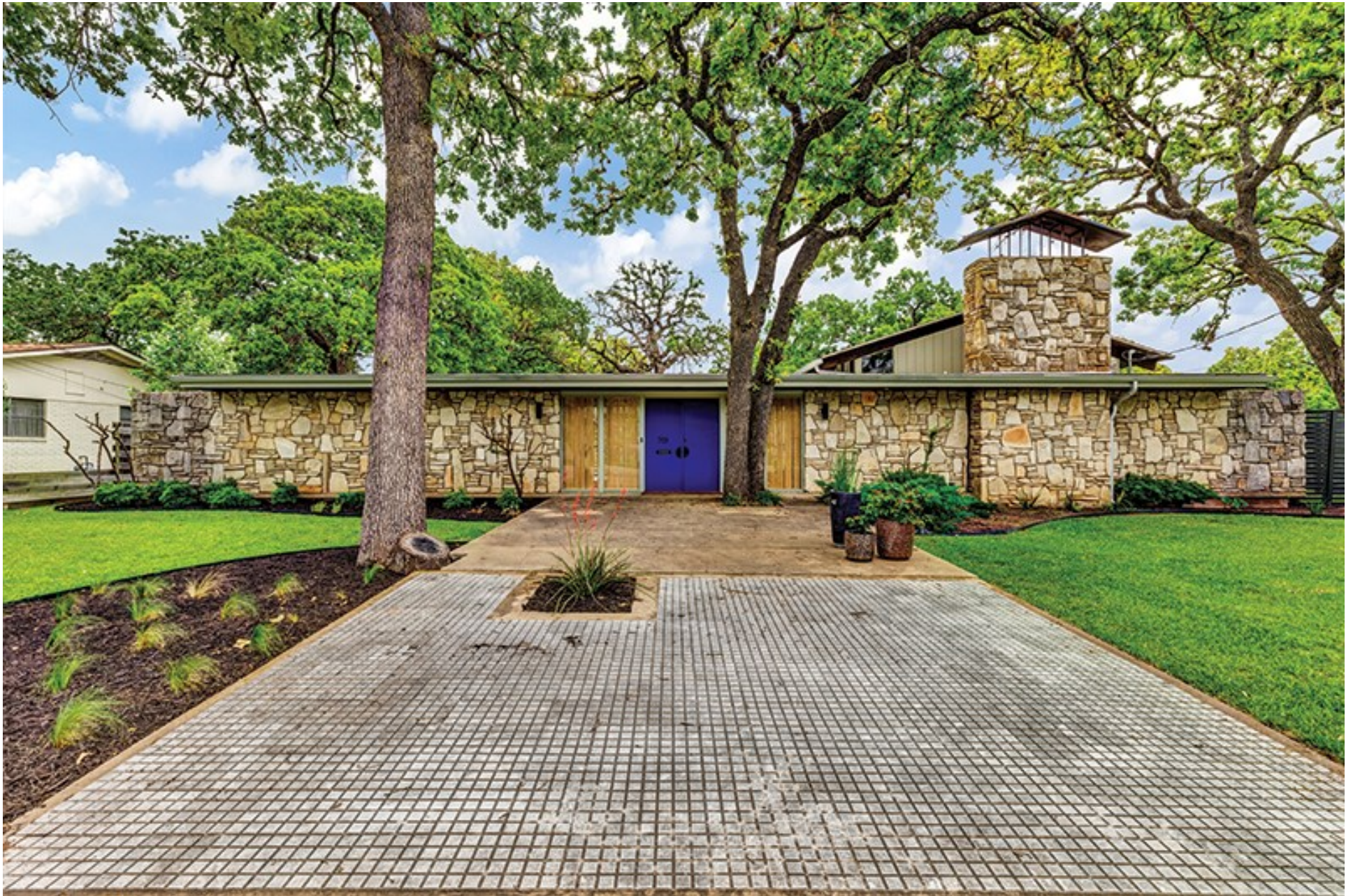
701 N. Milam—The Jack Stehling, AIA house
