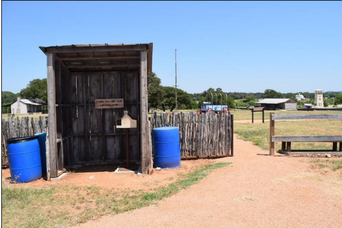
Figure B-3. West entrance to Fort Martin Scott grounds with wood-framed information kiosk, facing southeast.
