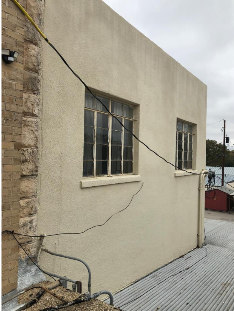
EAST VIEW OF CIRCA 1940'S ADDITION WHERE NEW STAIRWAY IS PLANNED
