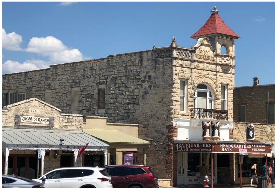
SOUTHWEST VIEW AT MAIN STREET
