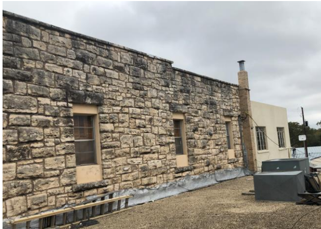
EAST SIDE VIEW OF BANK BUILDING LOOKING NORTH
