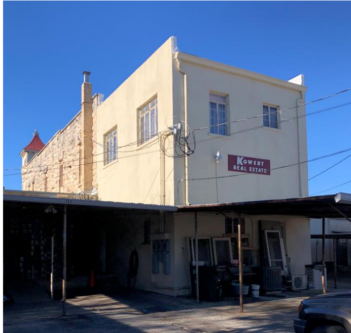
REAR VIEW OF BANK BUILDING WITH LATER ADDITION
