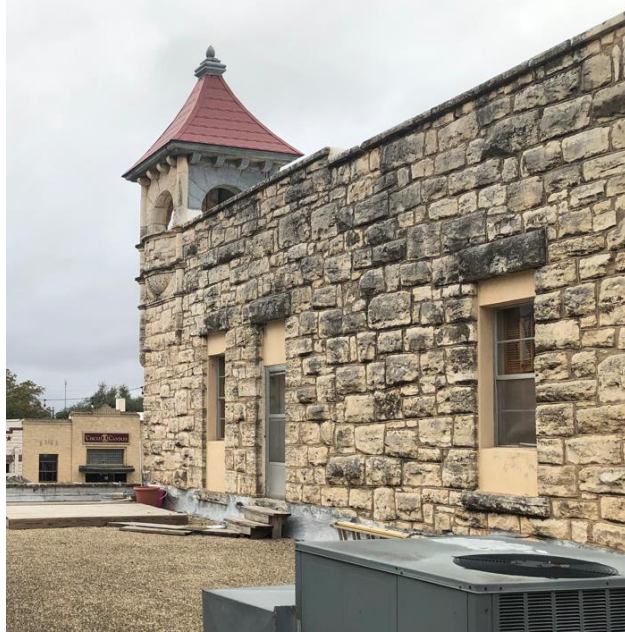
EAST SIDE VIEW OF BANK BUILDING LOOKING SOUTH
