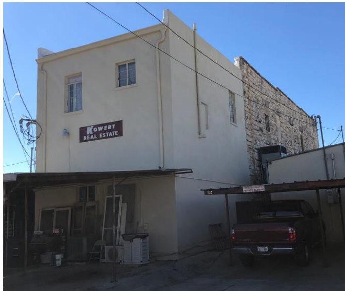
REAR NORTHWEST VIEW OF LATER ADDITION
