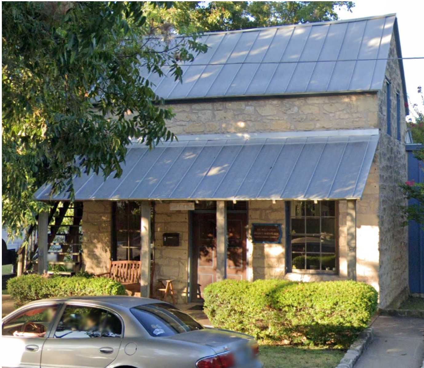
Existing Sunday House - North Elevation
