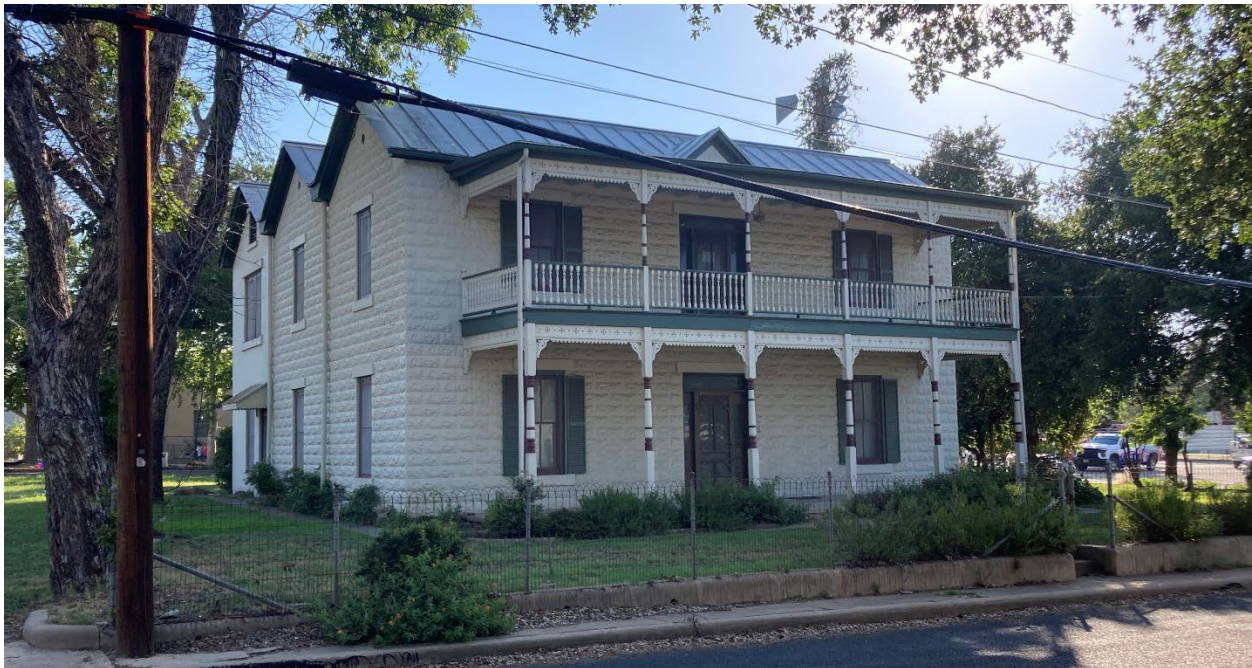
Southwest elevation looking northeast
