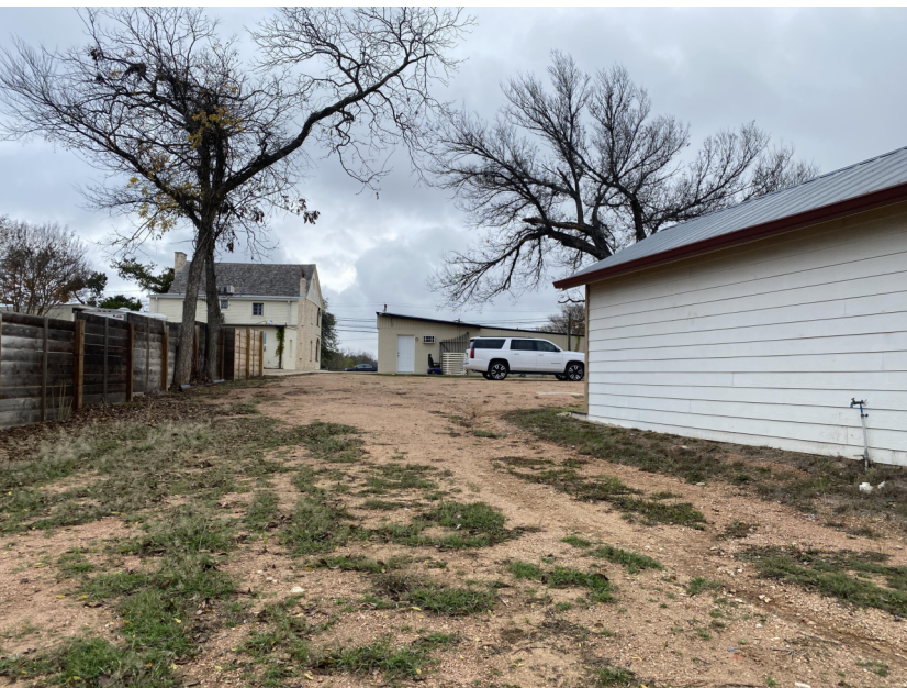
EXISTING UPPER CASITA
