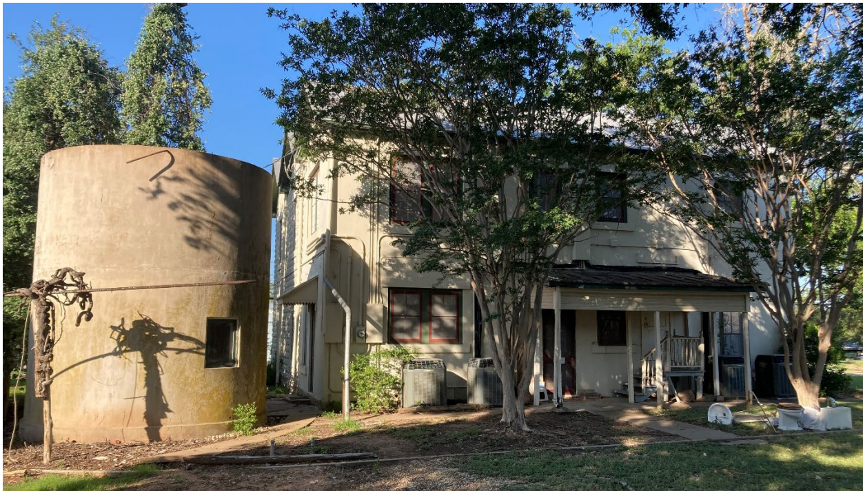
North elevation looking south
