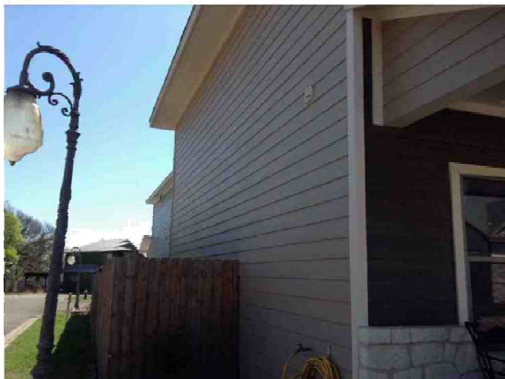
Side view NORTH VIEW
