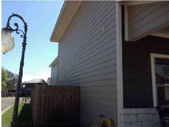
Side view NORTH VIEW
