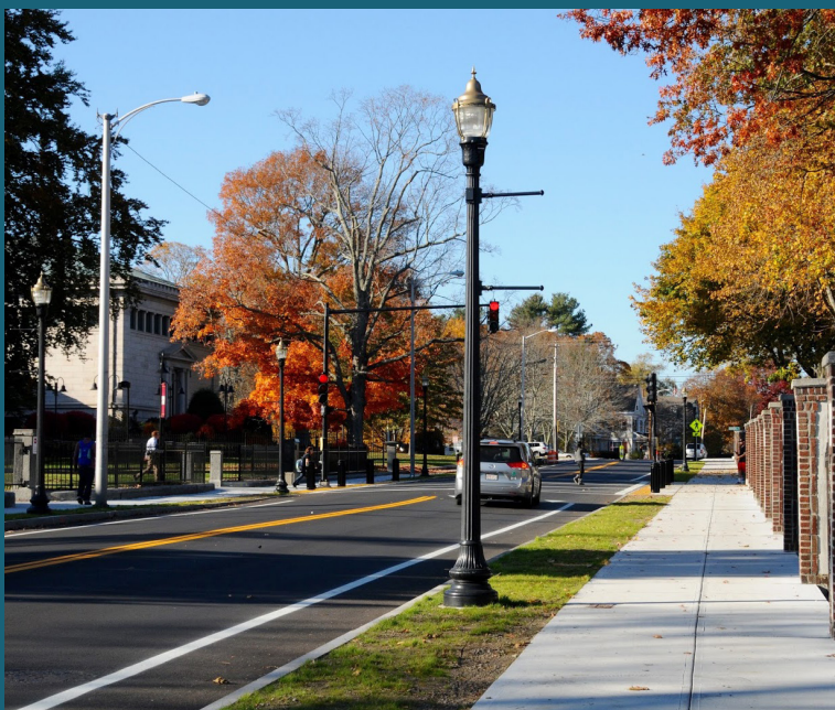
Streets with character can include elements such as sidewalks, lighting, and bike lanes. Photo source: Franklin Downtown Partnership
