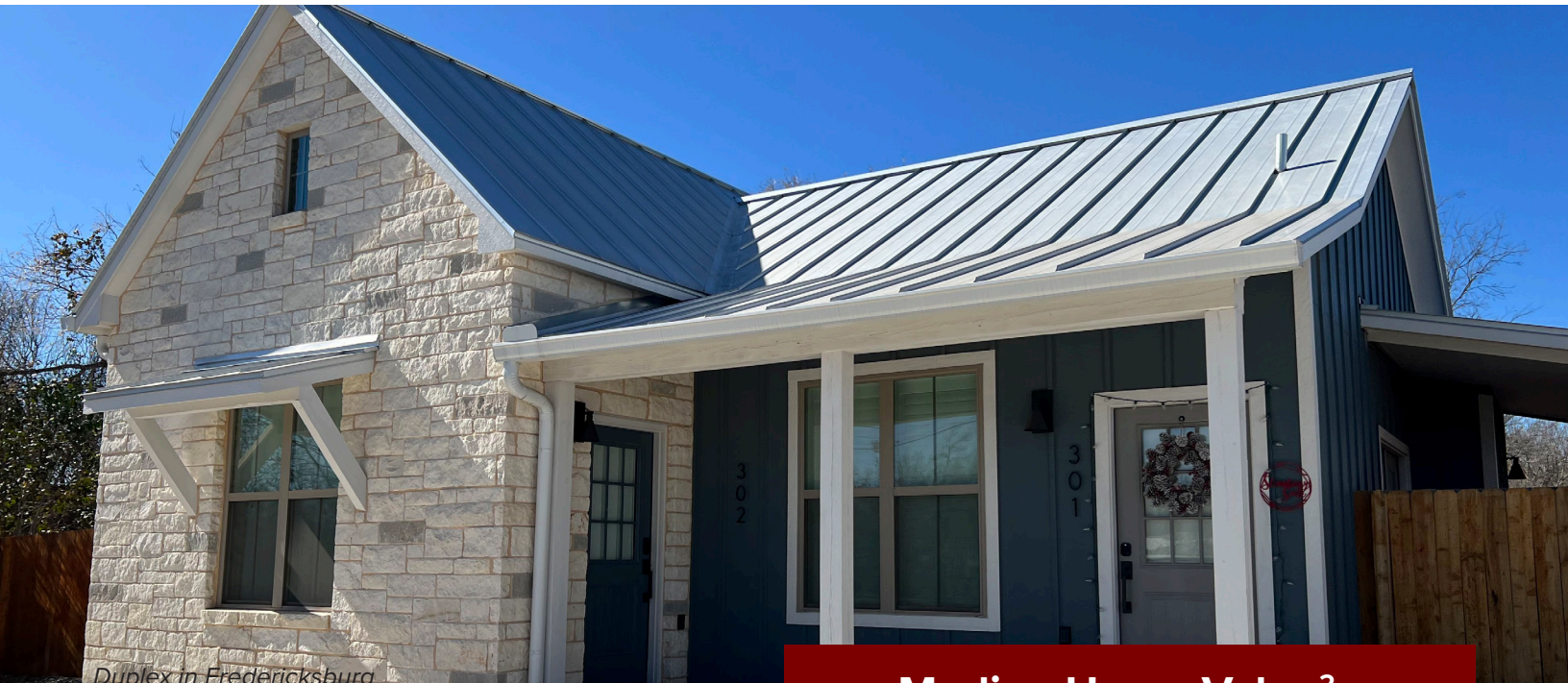
Duplex in Fredericksburg
