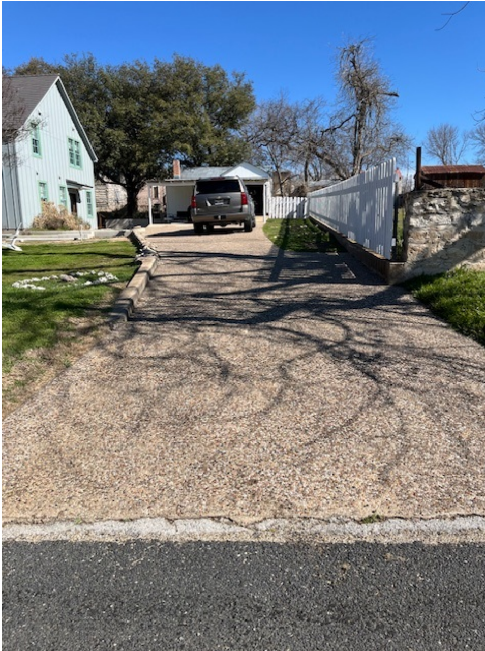
South East Side of Property – Driveway 10-12 Ft Wide – 48 Ft Long
