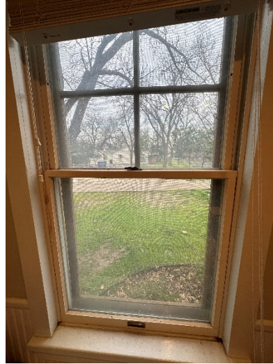
East side windows replaced in the 90's
