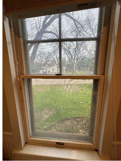
East side windows replaced in the 90's
