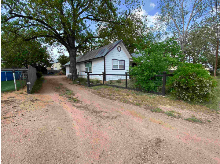
View from SW corner
