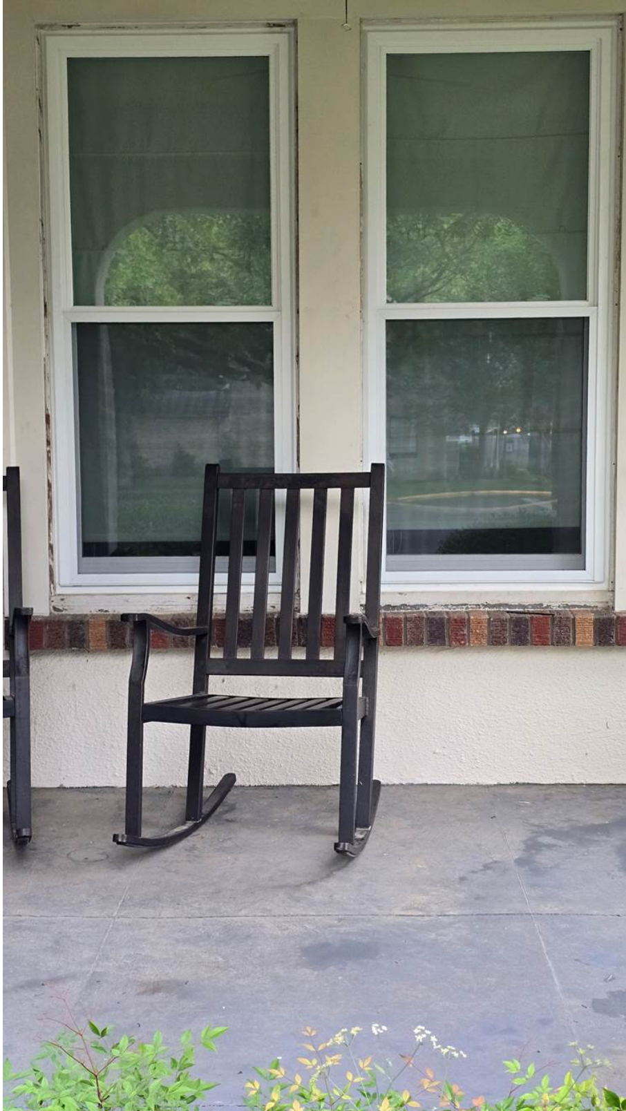
Wood windows replaced with Vinyl
