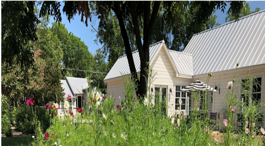
View of existing structure from southeast - post garden construction.
