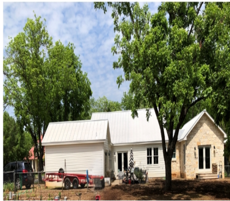
View of existing structure from south - during garden construction.
