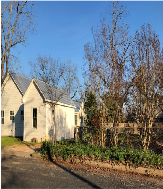
View of home from N. Lincoln. Workshop addition to be to the right (south) of structure.
