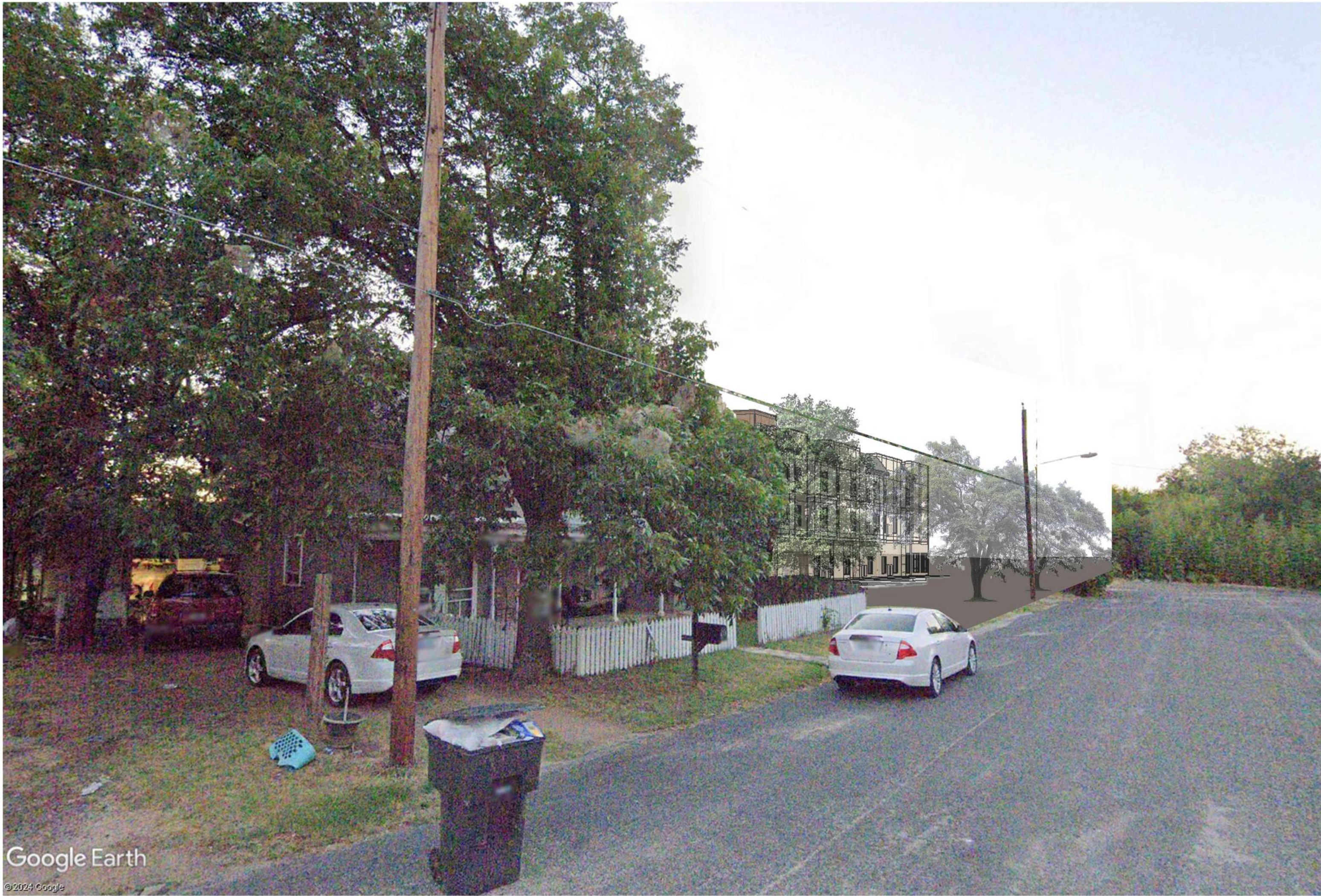
4 SP-3 VIEW FROM E. SAN ANTONIO ST.
