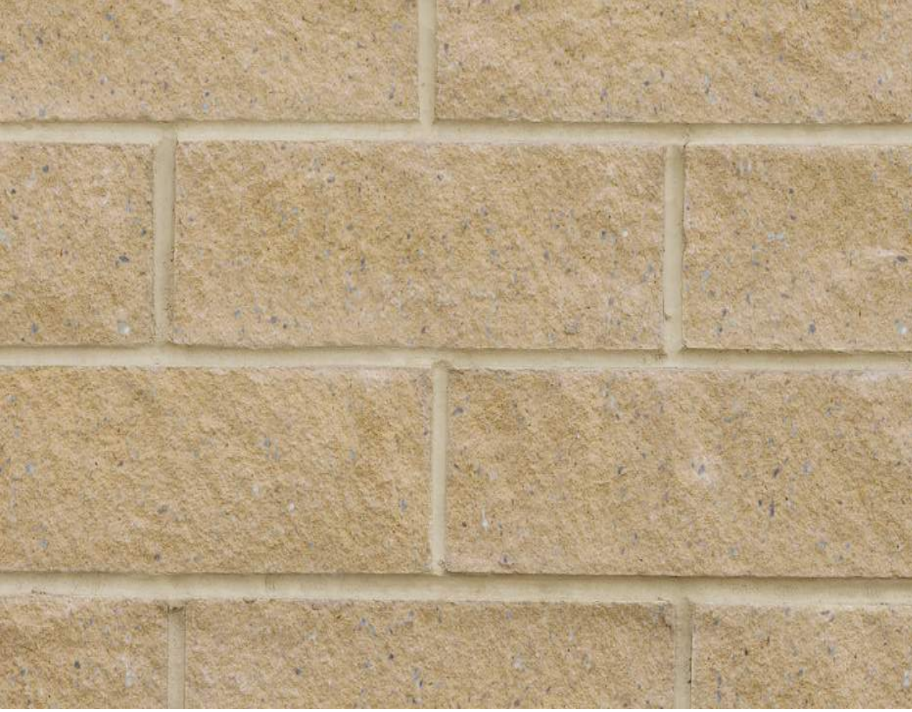
EXTERIOR PATIO/POOL WALL : SPLIT FACE CMU W/ STONE CAP
