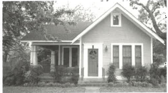
Figure 3-20. Example of a Craftsman bungalow at 707 W. Main Street. Note that the 2-inch horizontal wood siding and relationship of wall to window are character-defining features to be preserved. Source: CMEC Historic Resources Survey, 2019.
