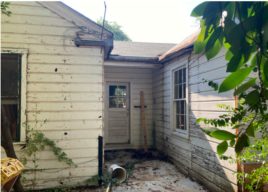
REAR (NORTHWEST ELEVATION) OF HOUSE TO BE PRESERVED GARAGE TO BE REMOVED ON LEFT
