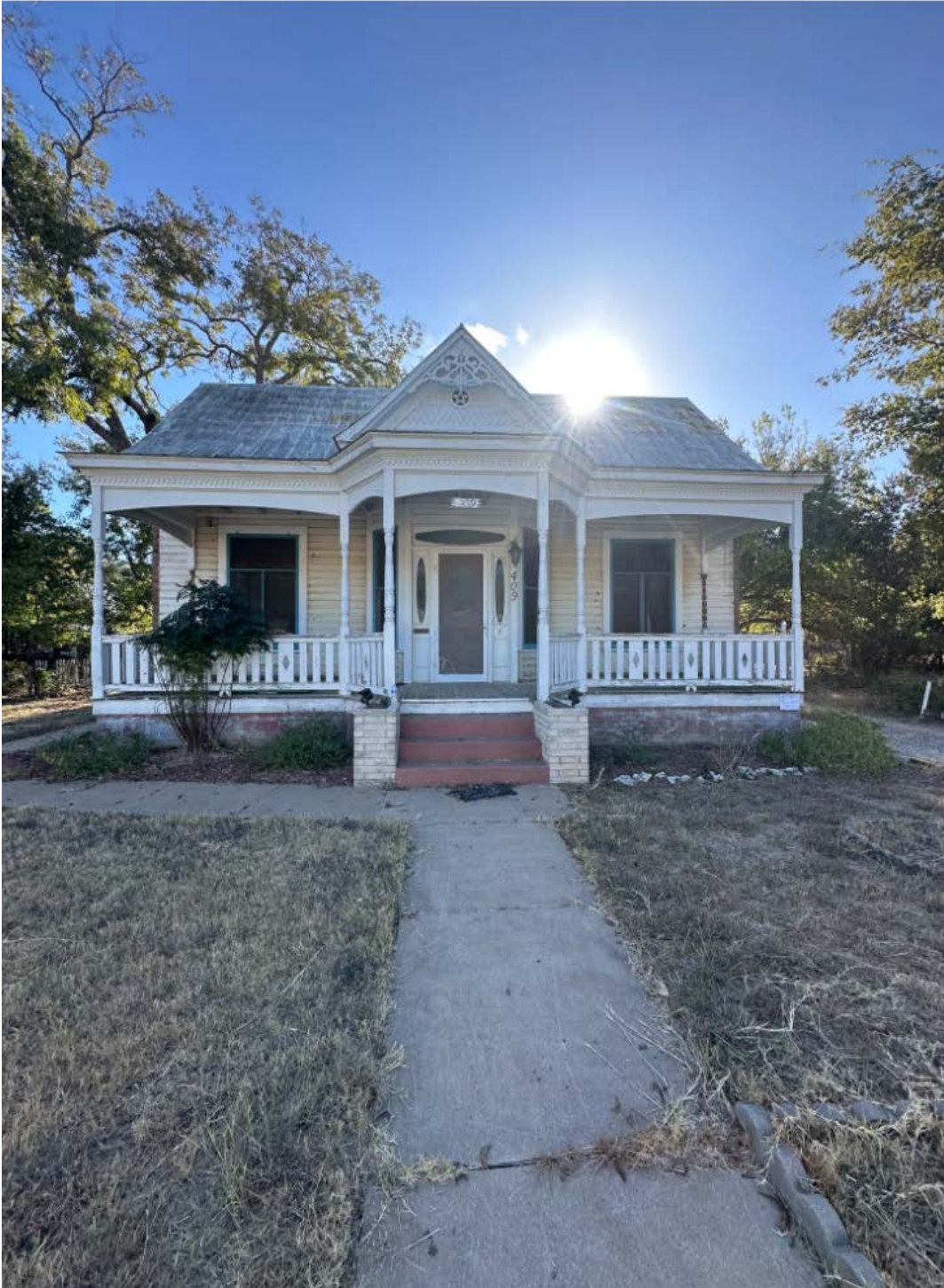
Front of Main Residence
