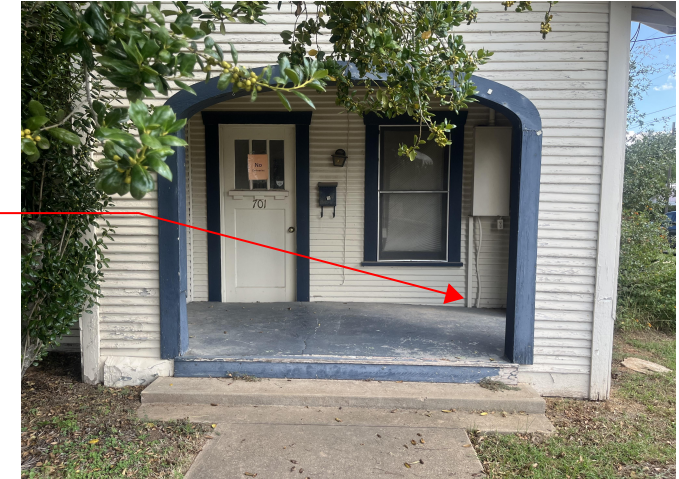
Figure 6: Front porch of 701 N. Llano St. facing Llano St. (2024)
