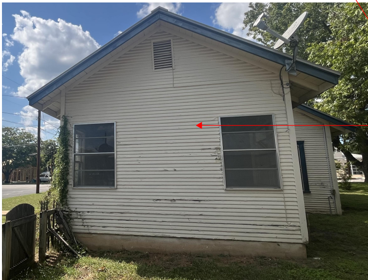
Figures 12: East Facade (2024)
