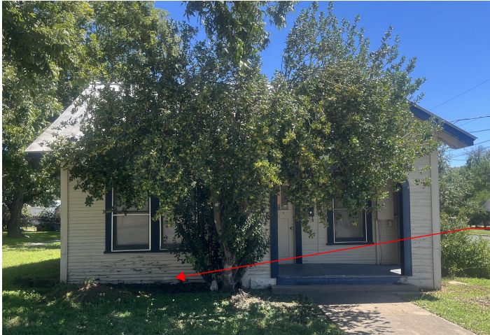
Figure 5: West facade of 701 N. Llano St. facing Llano St. (2024)
