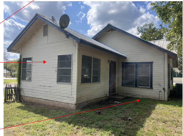
Figures 13: East Facade (2024)
