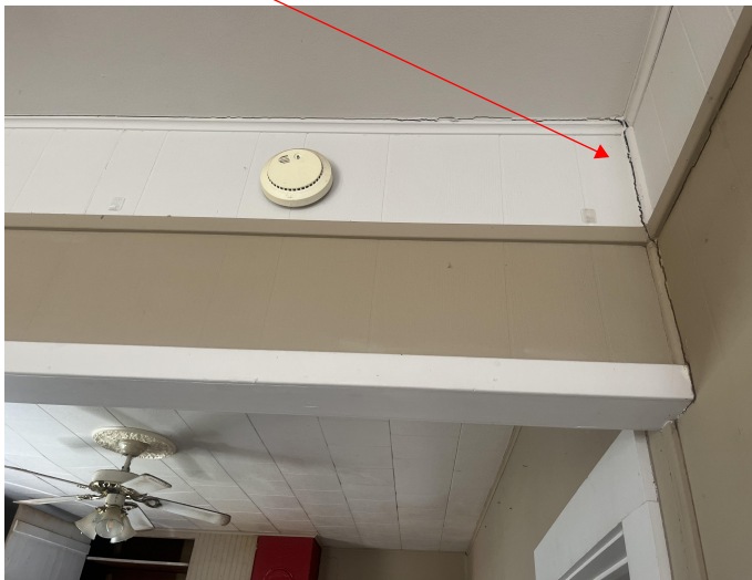
Figure 24: Beam between kitchen and addition (2024)
