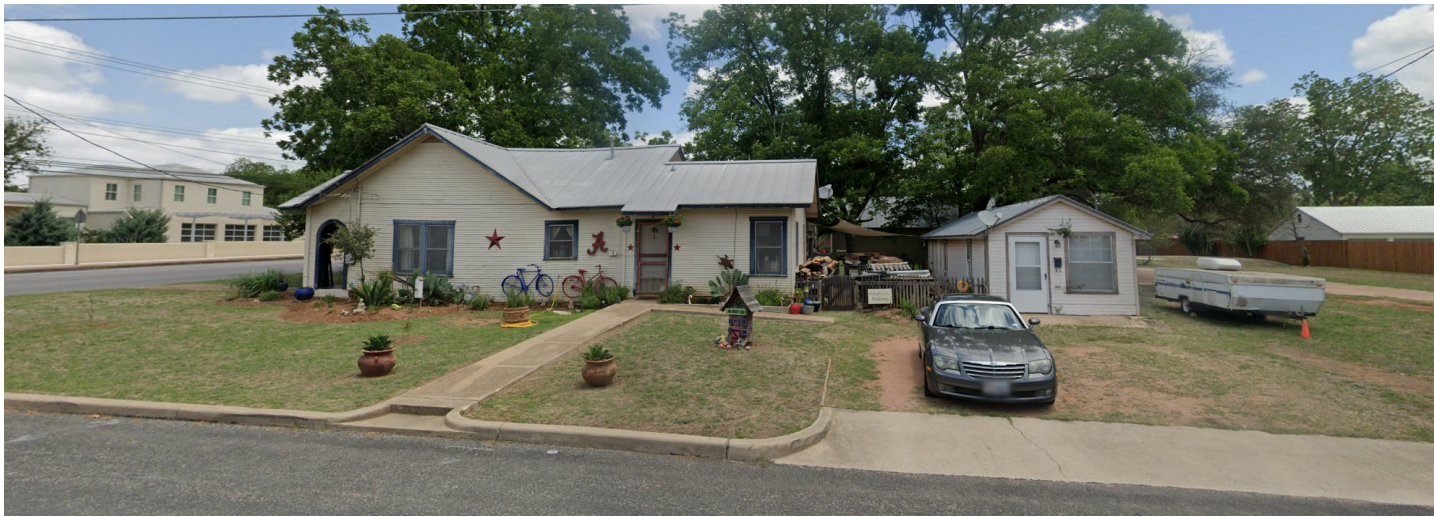
Figure 1: 701 N. Llano St. facing Centre St. (2024)
