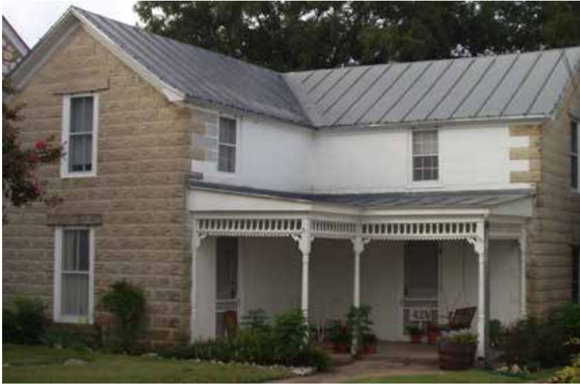
Figure 3-14. Example of original Folk Victorian porch detailing at 421 W. Main. Note how the turned porch posts are integrated into the masonry with attention to detail seldom replicated in non-historic examples. Source: HHM 2002 Survey.
