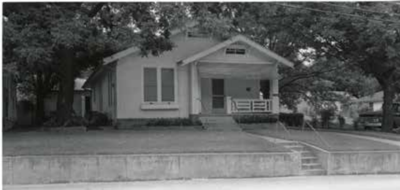
Figure 3-15. Example of original character-defining Craftsman-style porch detailing on a ca. 1920 bungalow at 308 E. San Antonio. Source: National Register Nomination, Fredericksburg Historic District, 1983.
