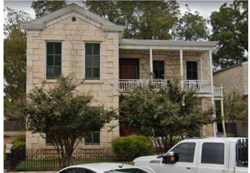
Figure 3-16. Example of an appropriate supplemental railing added above a historic balcony railing at 252 E. Main Street. Source: Google Street View.
