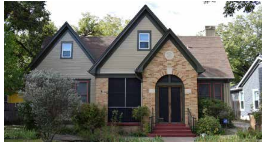
Figure 3-17. Example of a reversible porch screening that does not damage or obscure historic character-defining features, appropriate for Low or Medium priorities only . Source: HHM archives.
