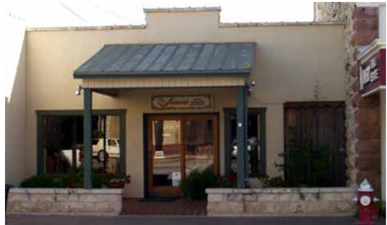
Figure 3-65. Example of an inappropriate ca. 1980 commercial building at 116 E. Main Street; its setback from the sidewalk interrupts the consistent line of storefronts. Source: HHM 2002 survey.
