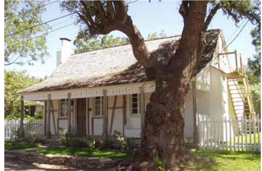
Figure 2-3. Photo of fachwerk construction at 512 W. Creek Street. Note the horizontal, vertical, and diagonal framing members. Also note the stucco finish and exterior stair. Source: HHM 2003 Historic Resources Survey.
