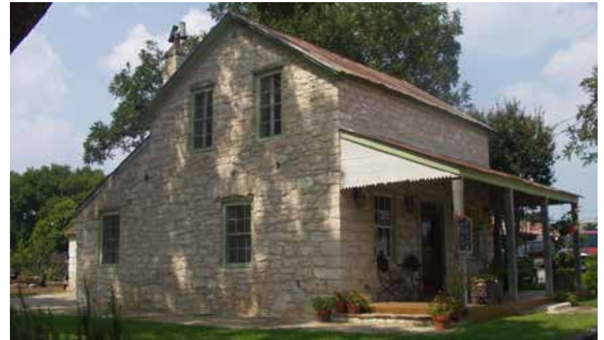
Figure 2-4. Photo of a limestone masonry vernacular house at 206 S. Adams Street. Note the arched lintels at the ground floor. Source: HHM 2003 Historic Resources Survey.
