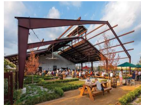
EXPOSED PEMB STRUCTURE
