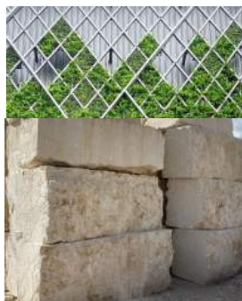
GREEN + LIMESTONE BLOCK SCREEN @ HWY 87
