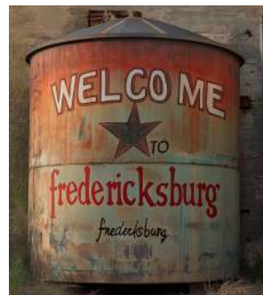
PAINTED BRANDING EXAMPLE ON CISTERN
