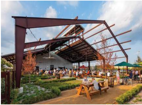
EXPOSED PEMB STRUCTURE
