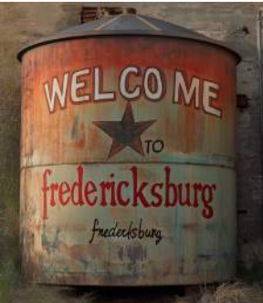
PAINTED BRANDING EXAMPLE ON CISTERN
