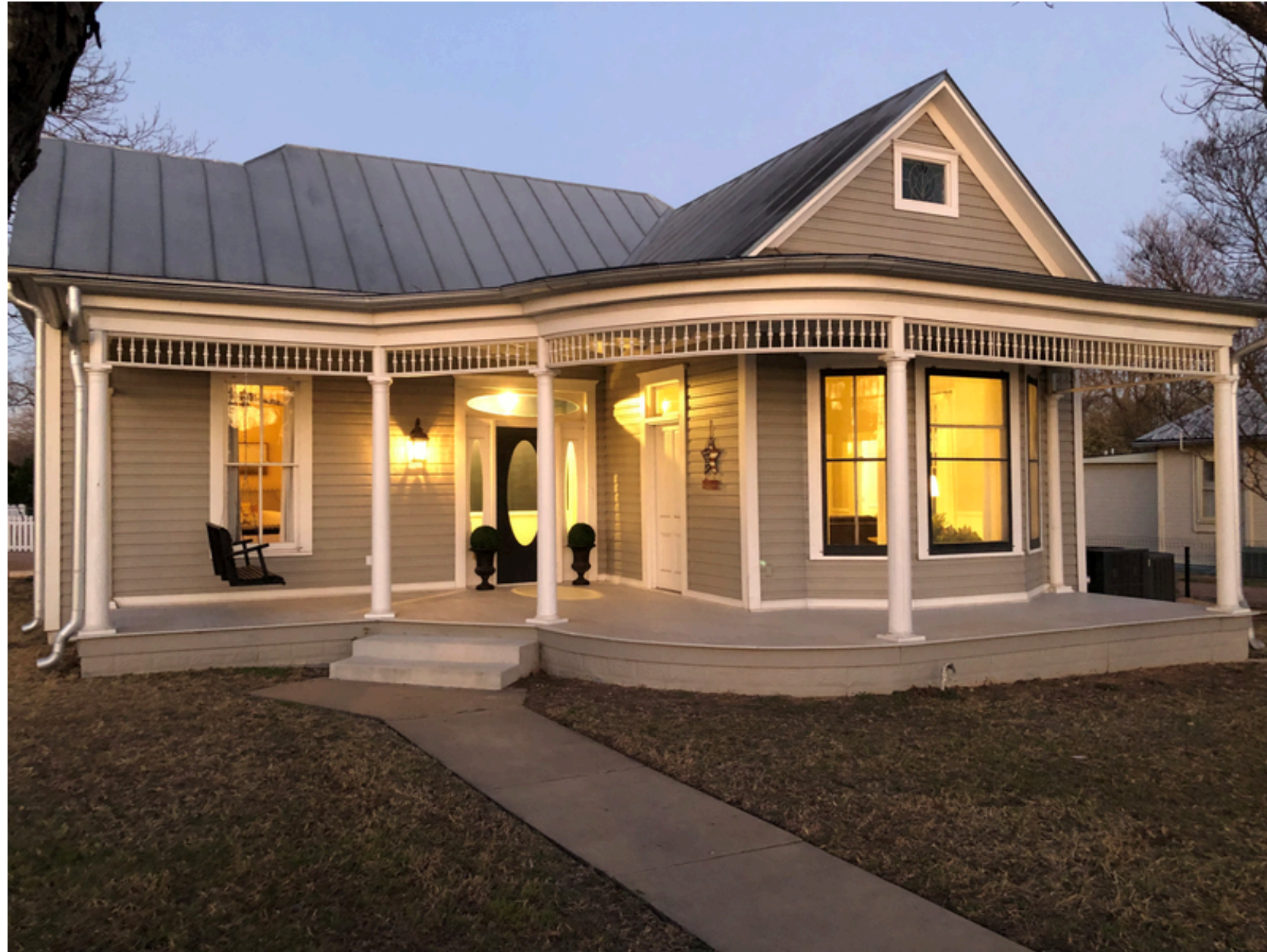
FRONT VIEW FROM E. TRAVIS
