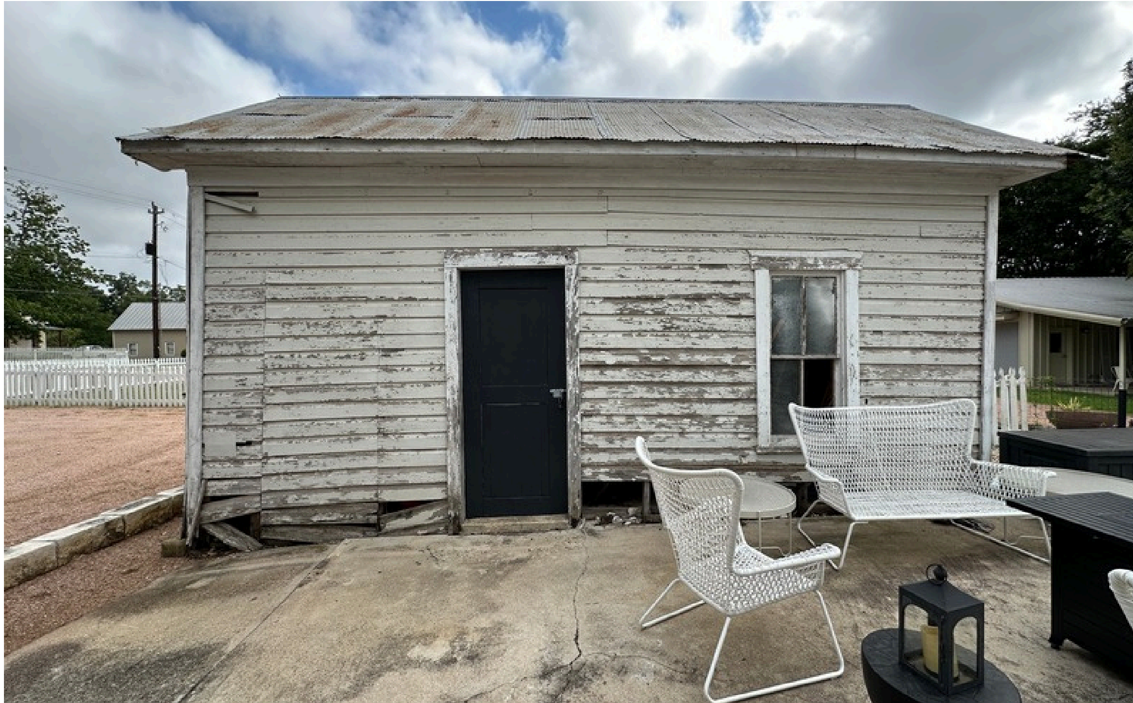
FULL VIEW OF SHED FROM THE HOUSE
