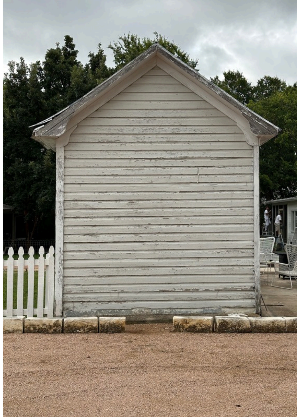
VIEW OF SHED FROM N WASHINGTON
