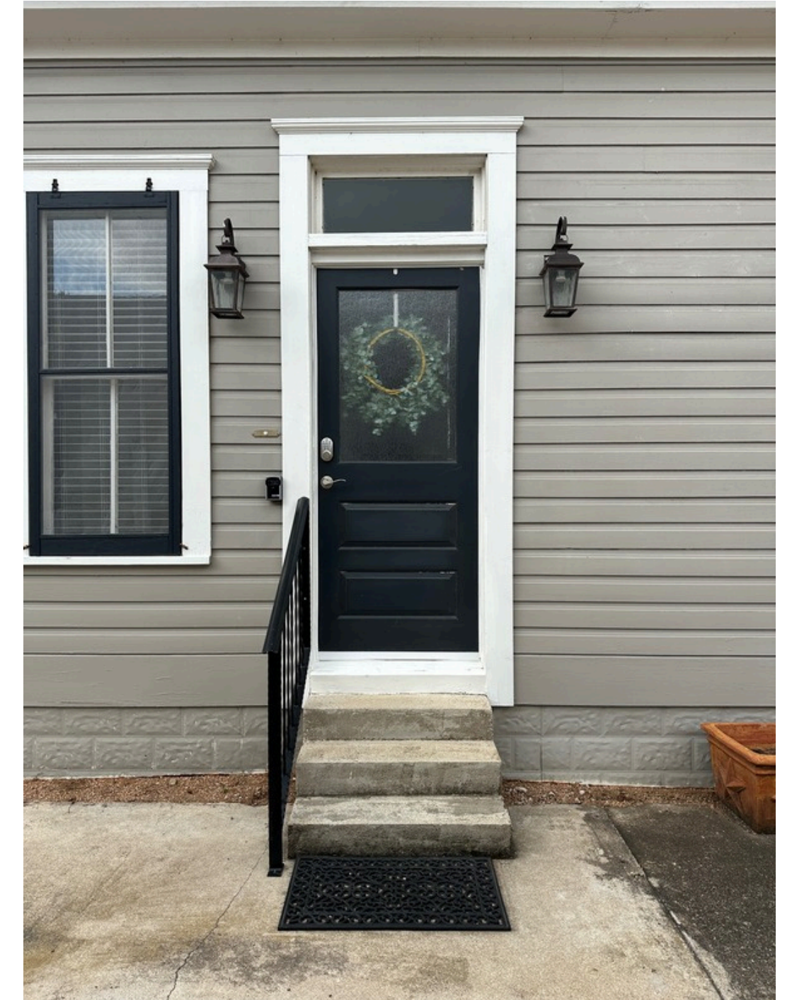
VIEW OF BACK PORCH
