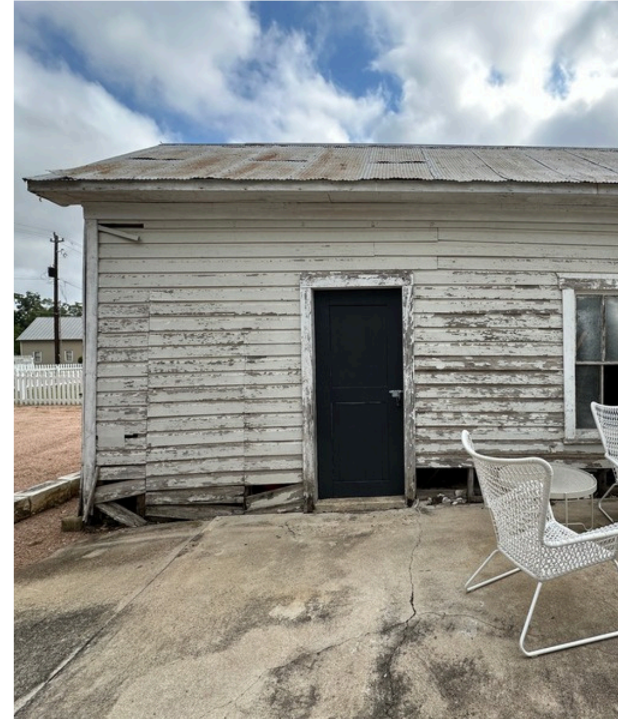
VIEW OF SHED FROM THE HOME
