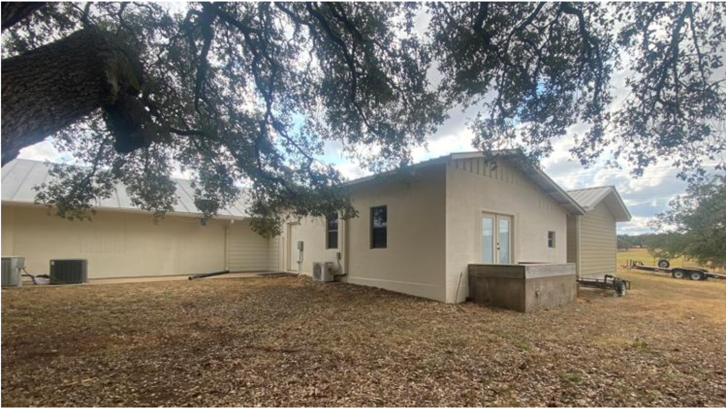
North (West Wing) View of Main Building
