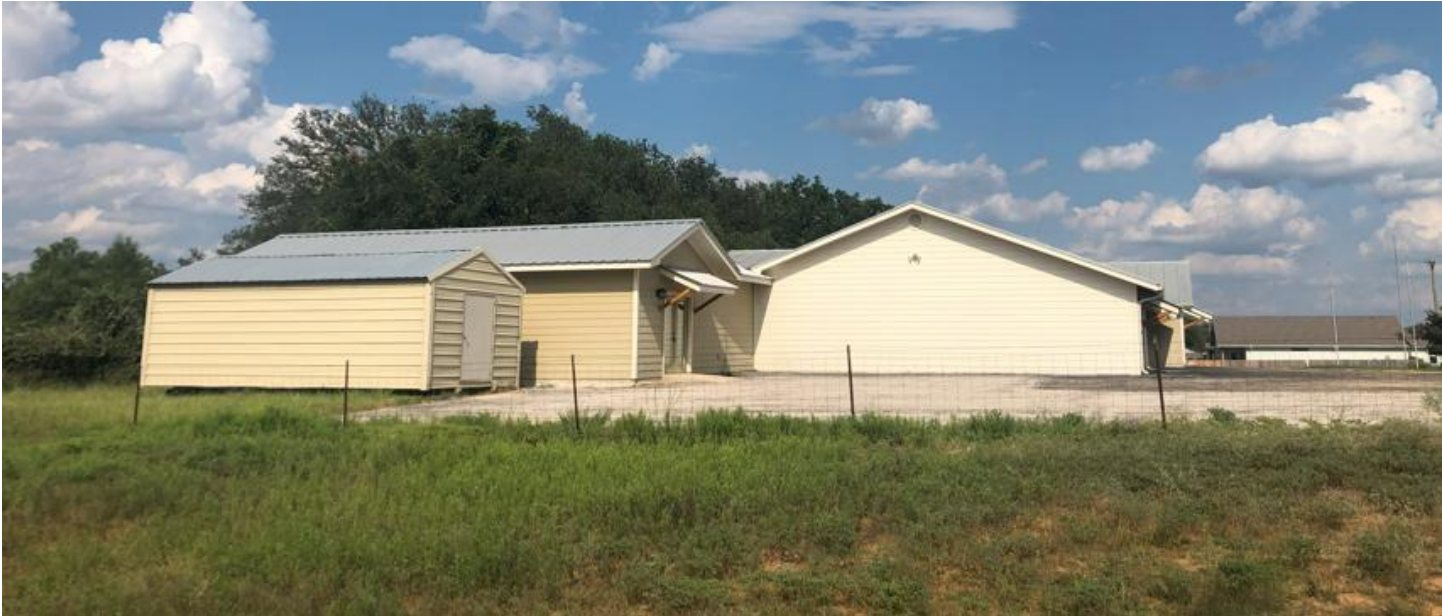
West Elevation of Main Building
