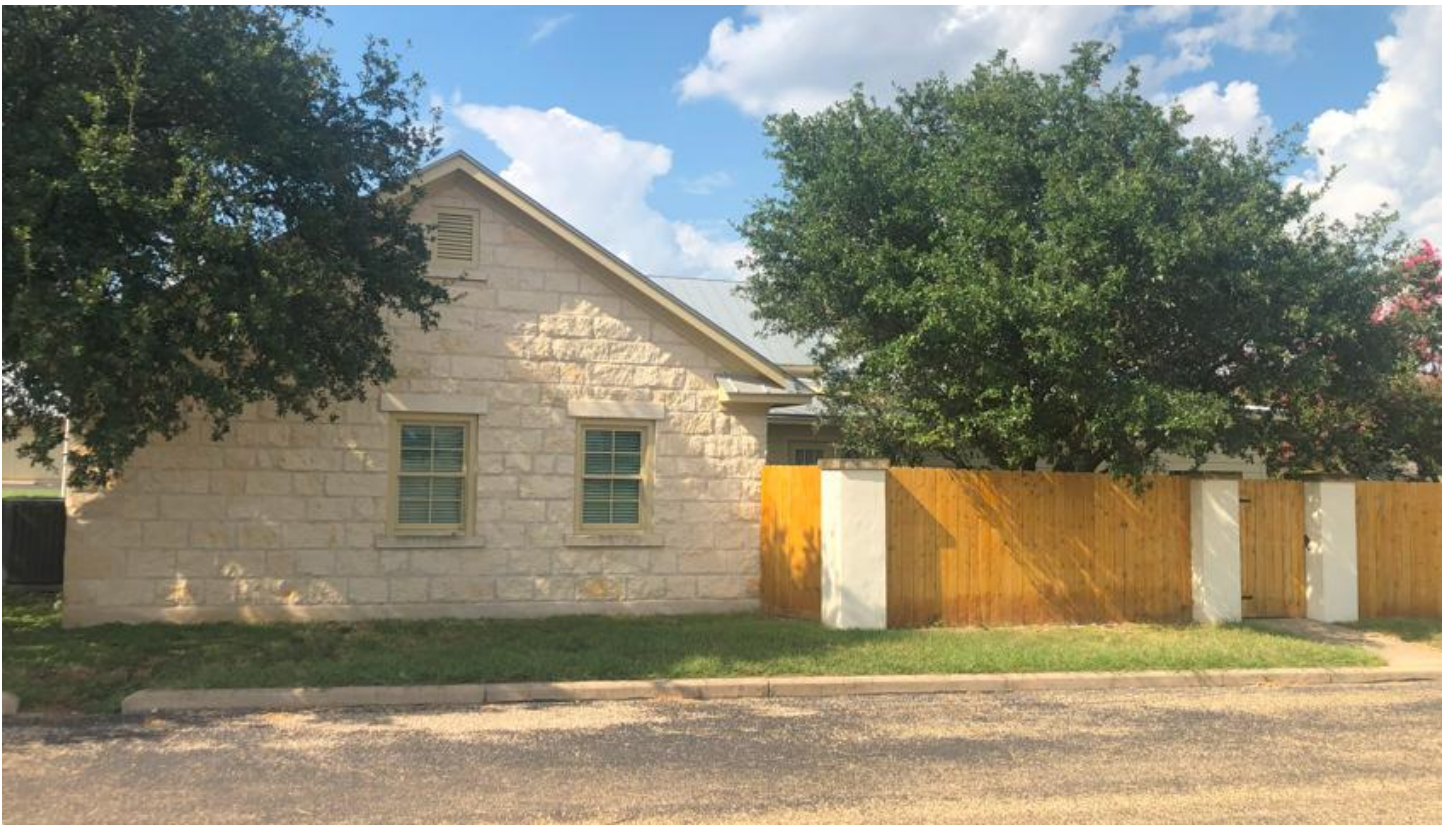
South Elevation of Cottage (No Work)
