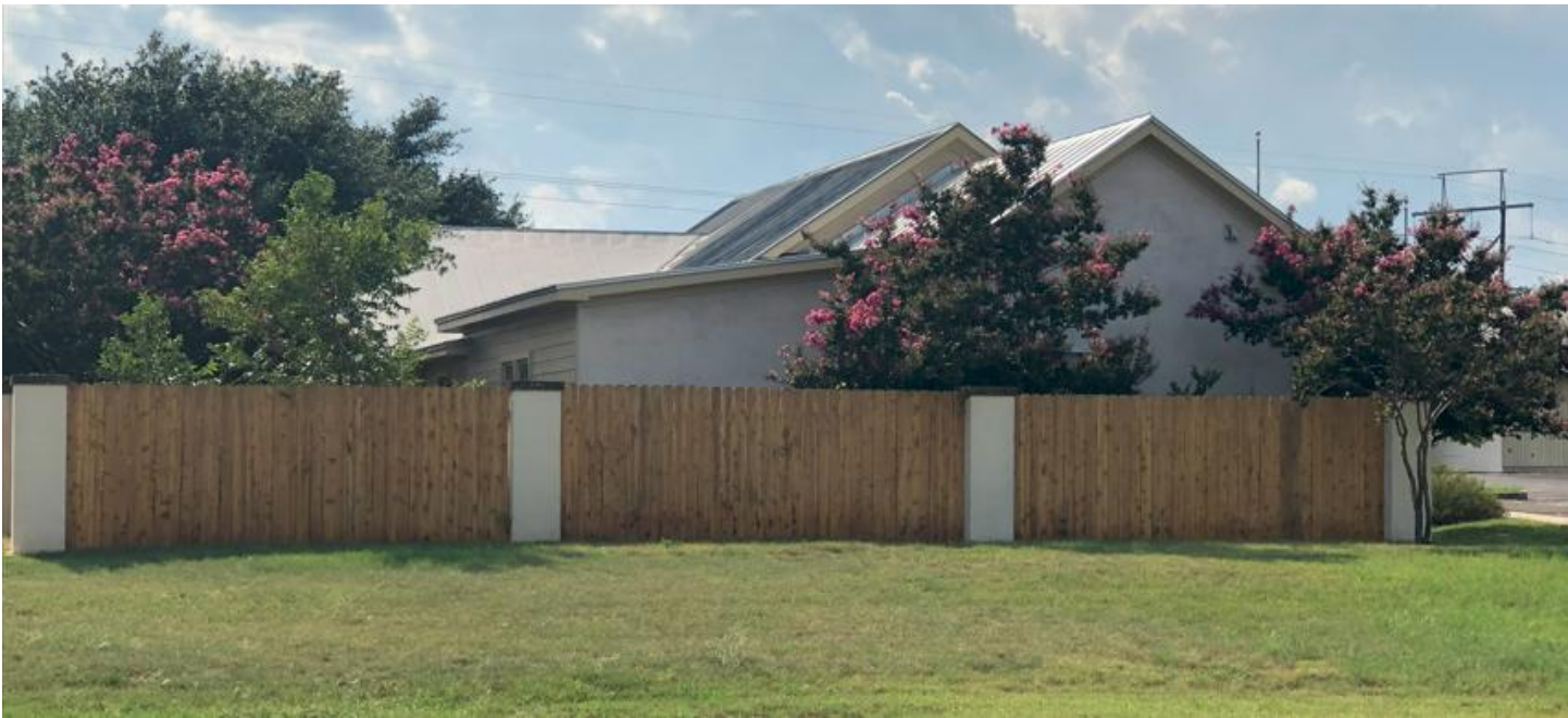
East Elevation of Cottage (No Work)
