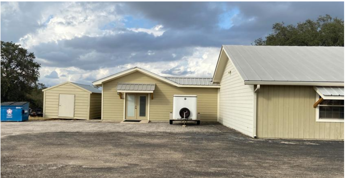
South Elevation of West addition
