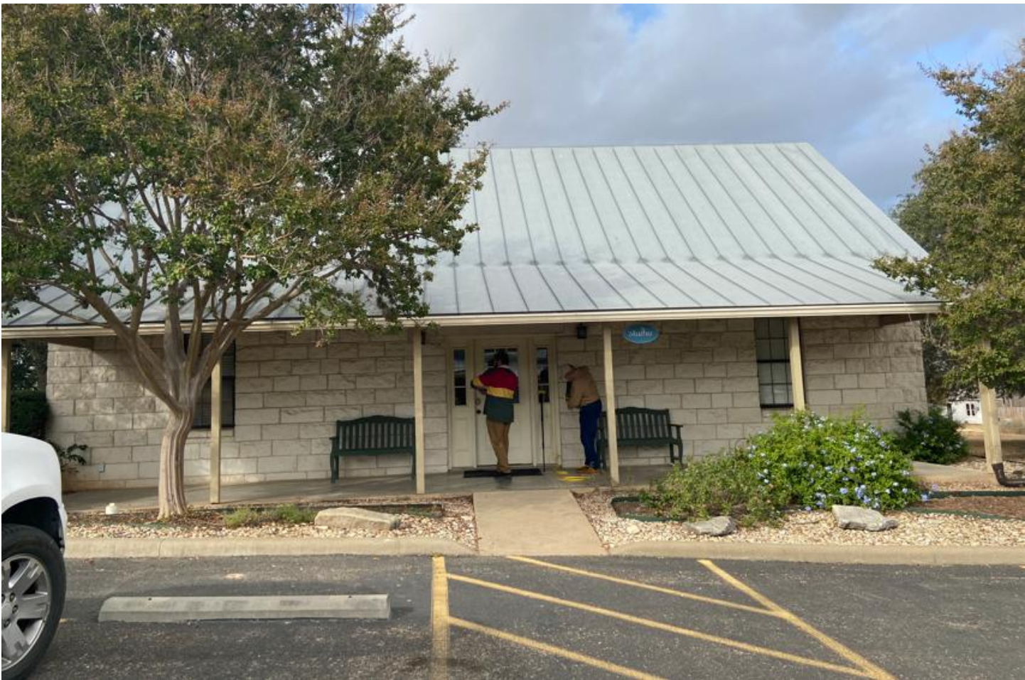
South Elevation of Existing Annex (East Wing) Building
