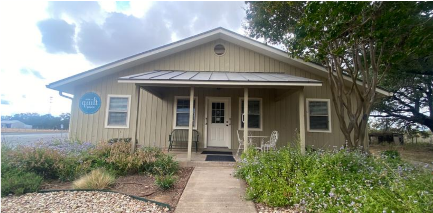
East Elevation of Main Building
