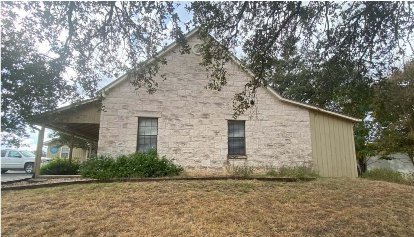
East Elevation of Existing Annex Building
