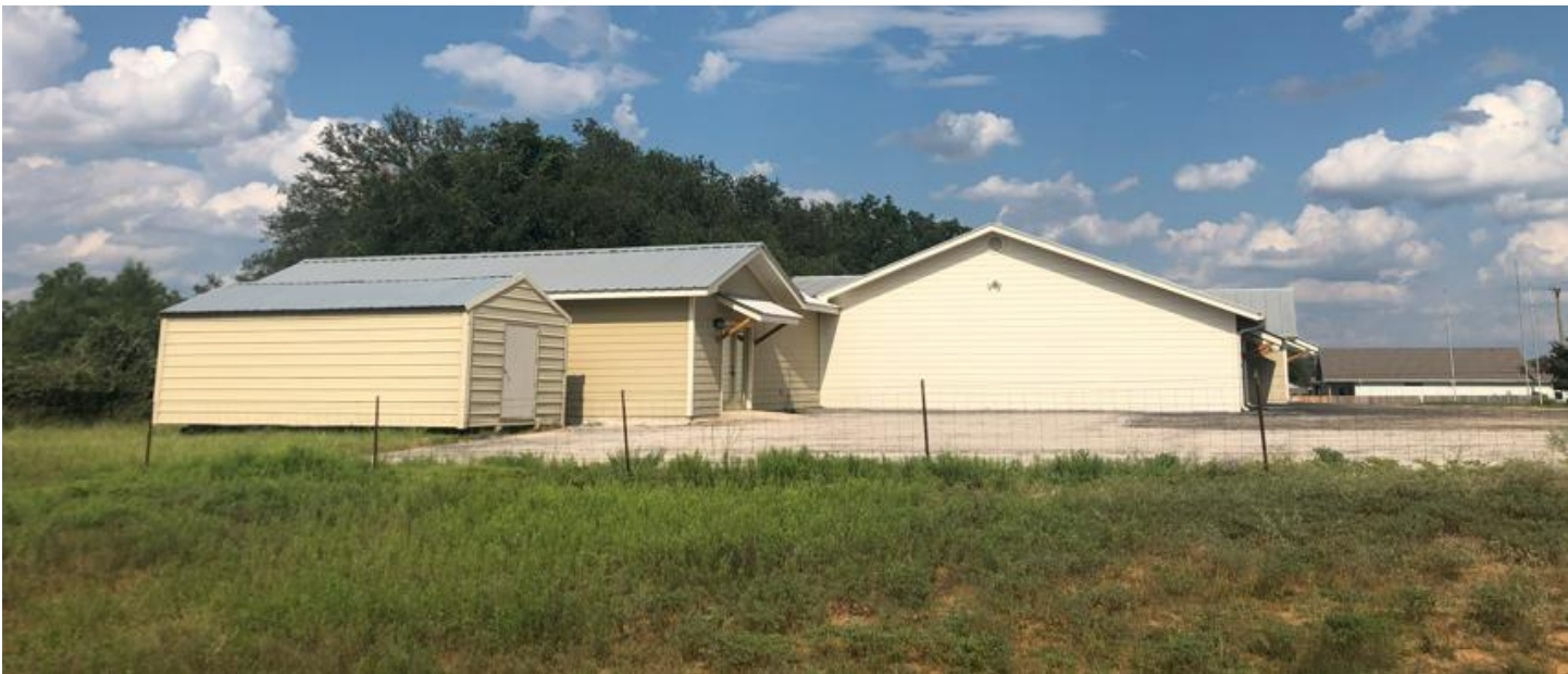
West Elevation of Main Building
