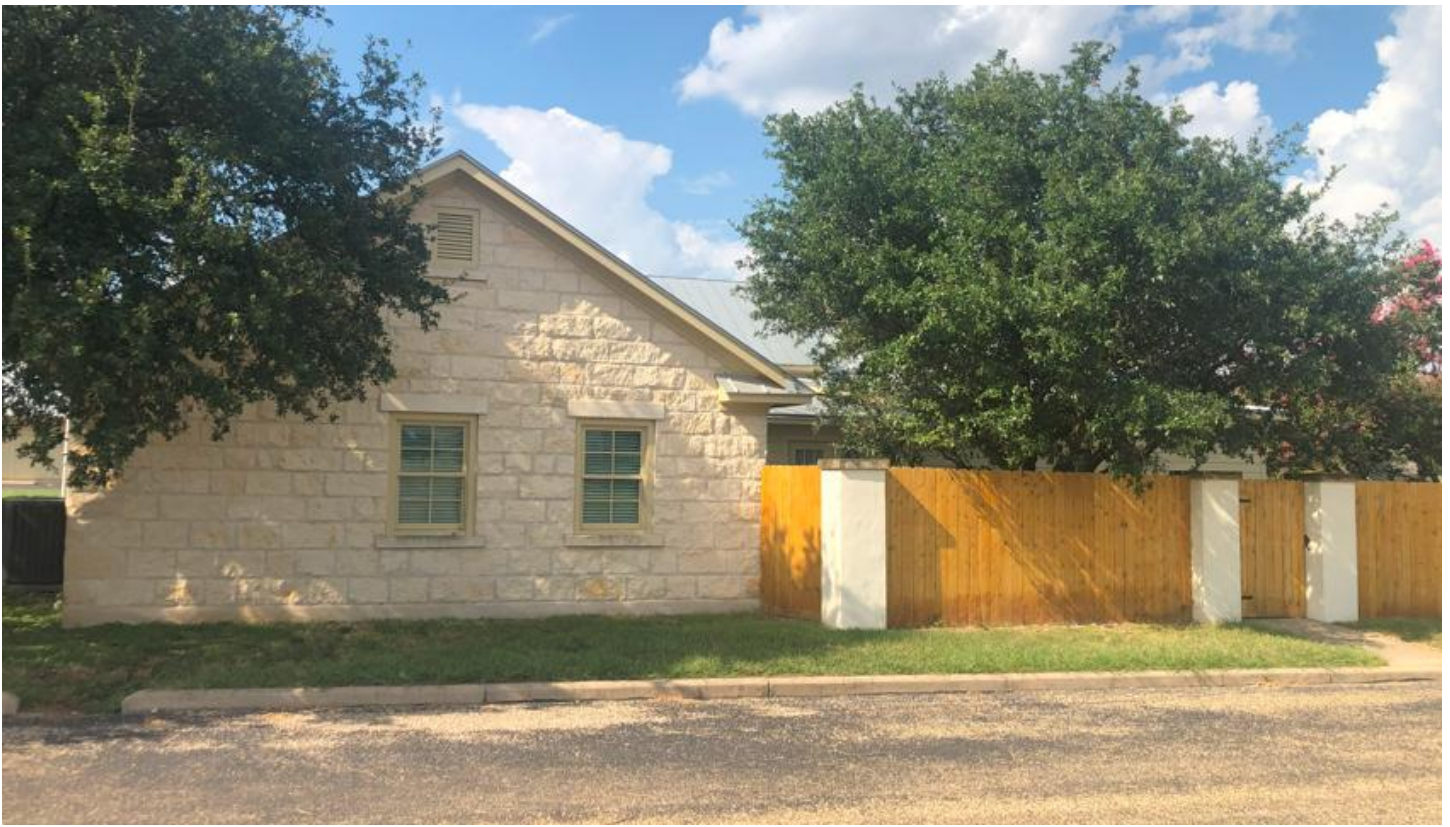
South Elevation of Cottage (No Work)
