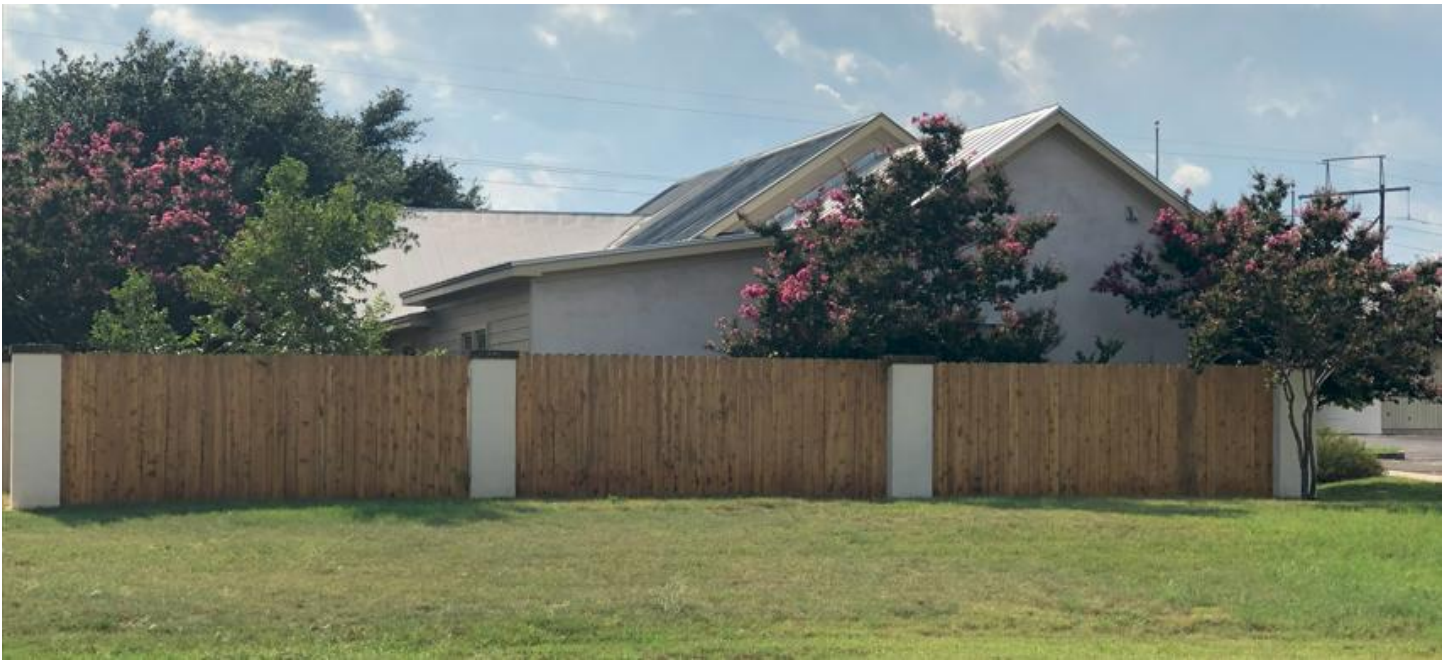
East Elevation of Cottage (No Work)
