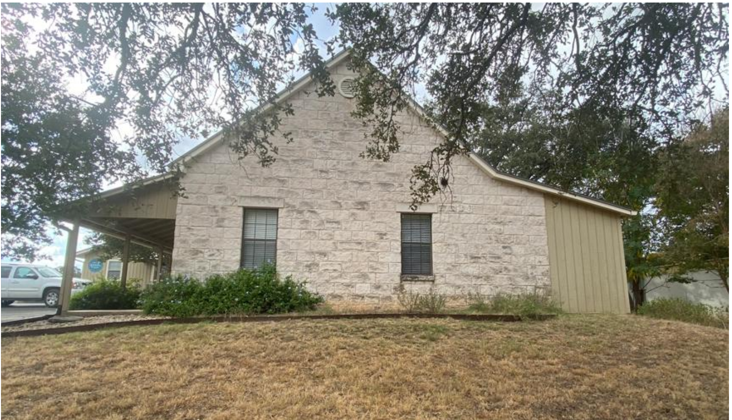
East Elevation of Existing Annex Building
