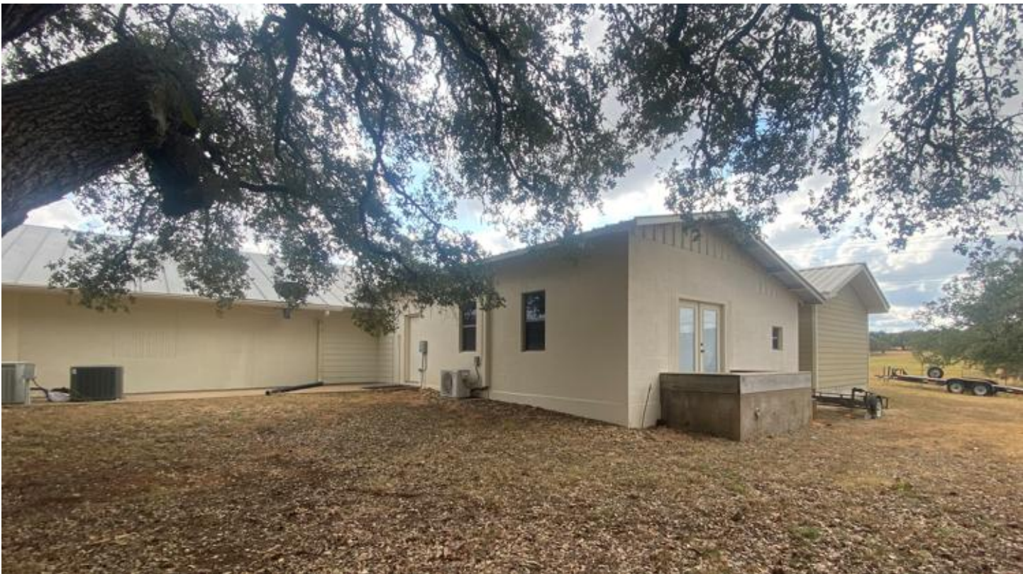
North (West Wing) View of Main Building
