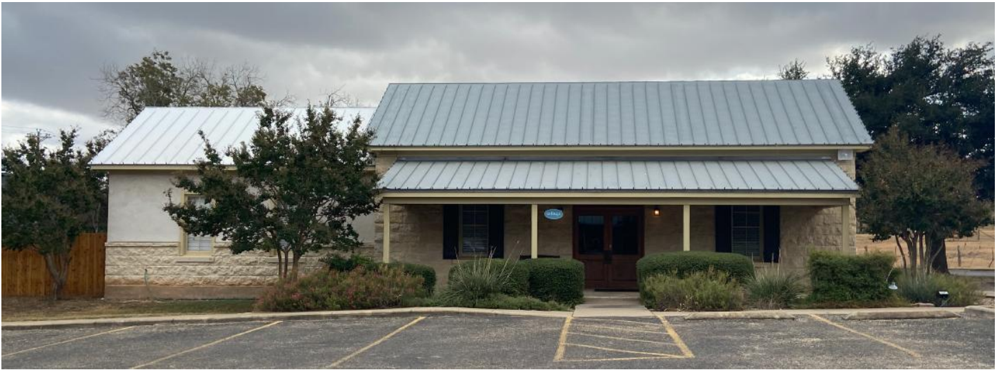
North Elevation of Existing Cottage (NO WORK)
