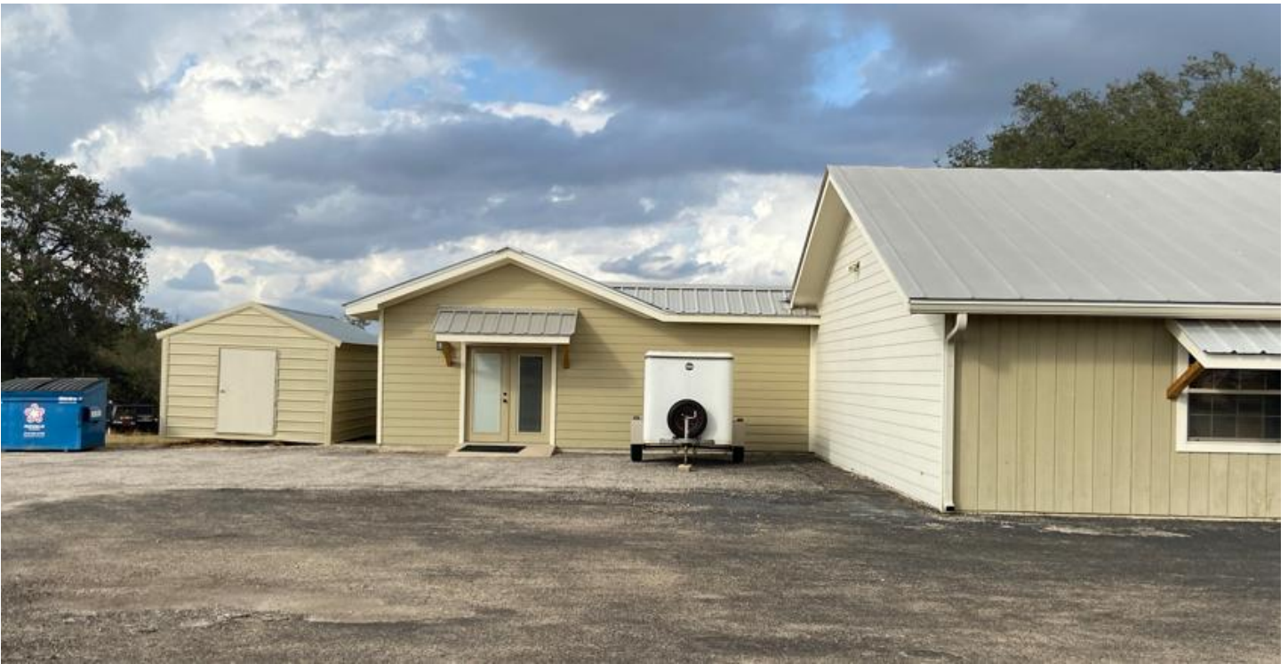
South Elevation of West addition
