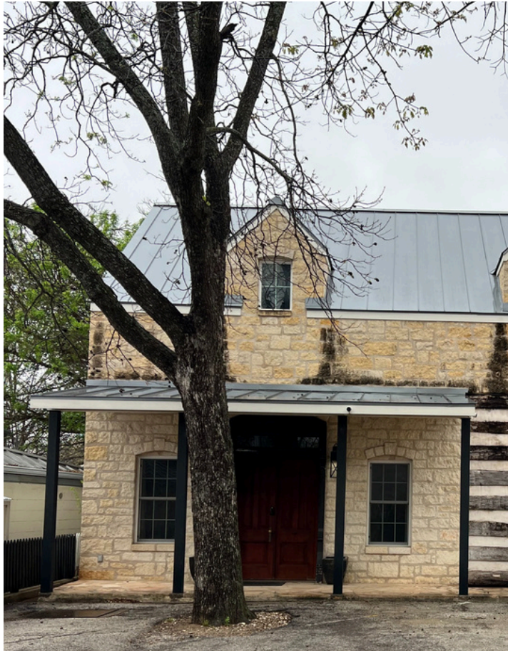
Existing Porch at entry of Guest House
