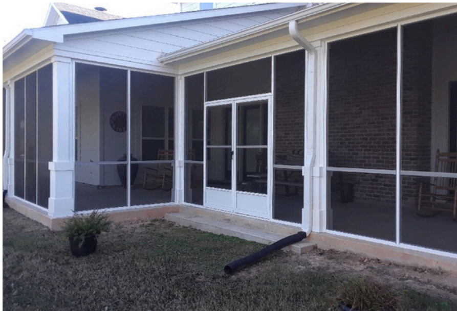
A second example from the designer shown to demonstrate a double door on a screened porch.
