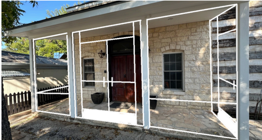
The mock-up of the screened porch over an image of the actual guest house porch.
