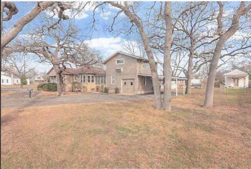
This is 707 N. Milam showing the main house, garage apartment and school house in back of the property
