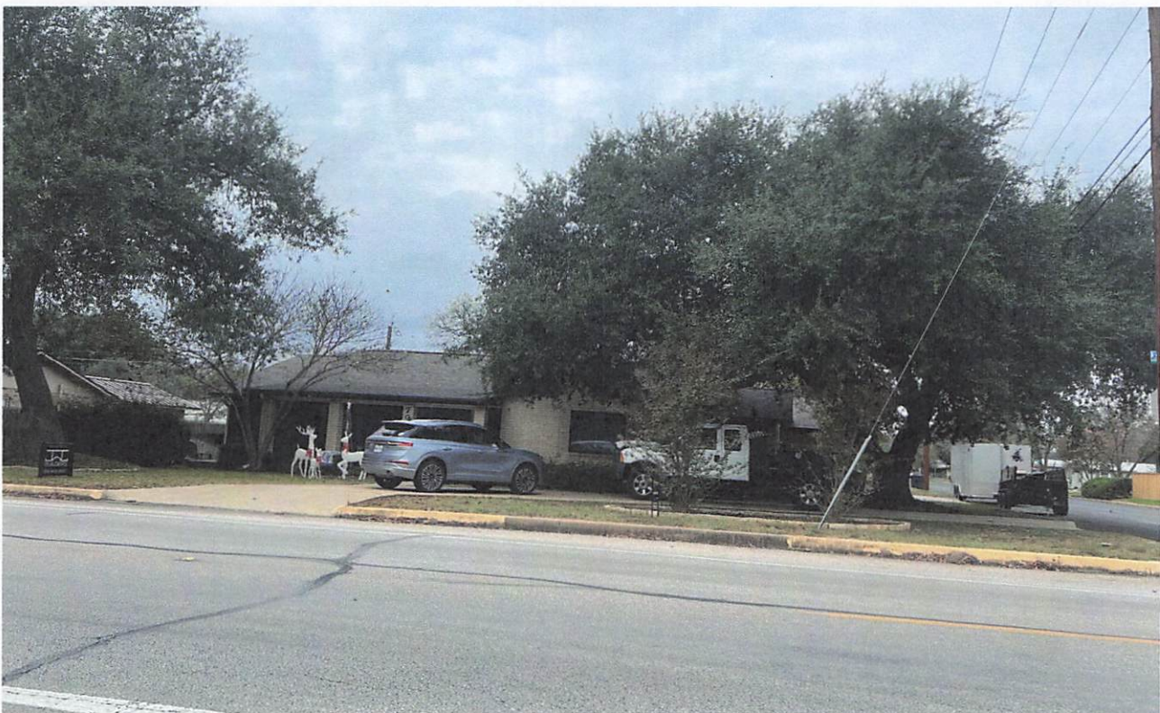
This is 710 N. Milam with signs showing "Home Builder" and "Powerhaus Electric"
