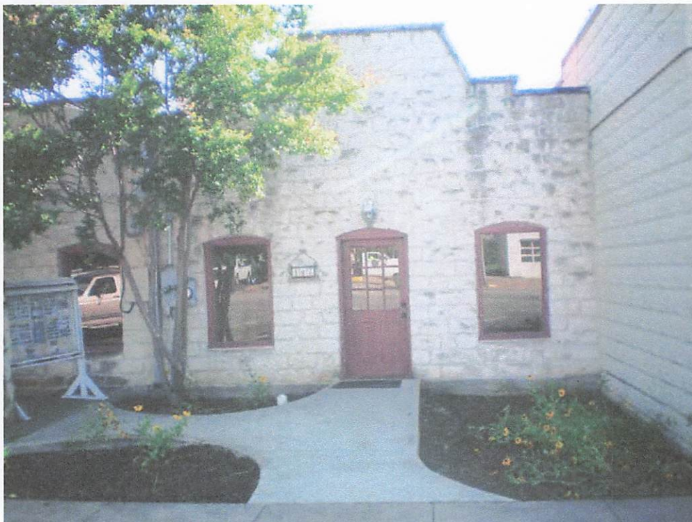
FRONT DETAIL OF 408 W. MAIN OFFICE
