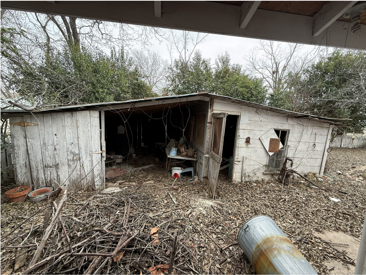
EXISTING SHED - PROPOSED TO BE DEMOLISHED
