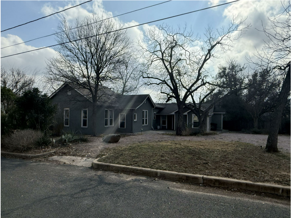
NEIGHBORING RESIDENCE TO THE EAST
