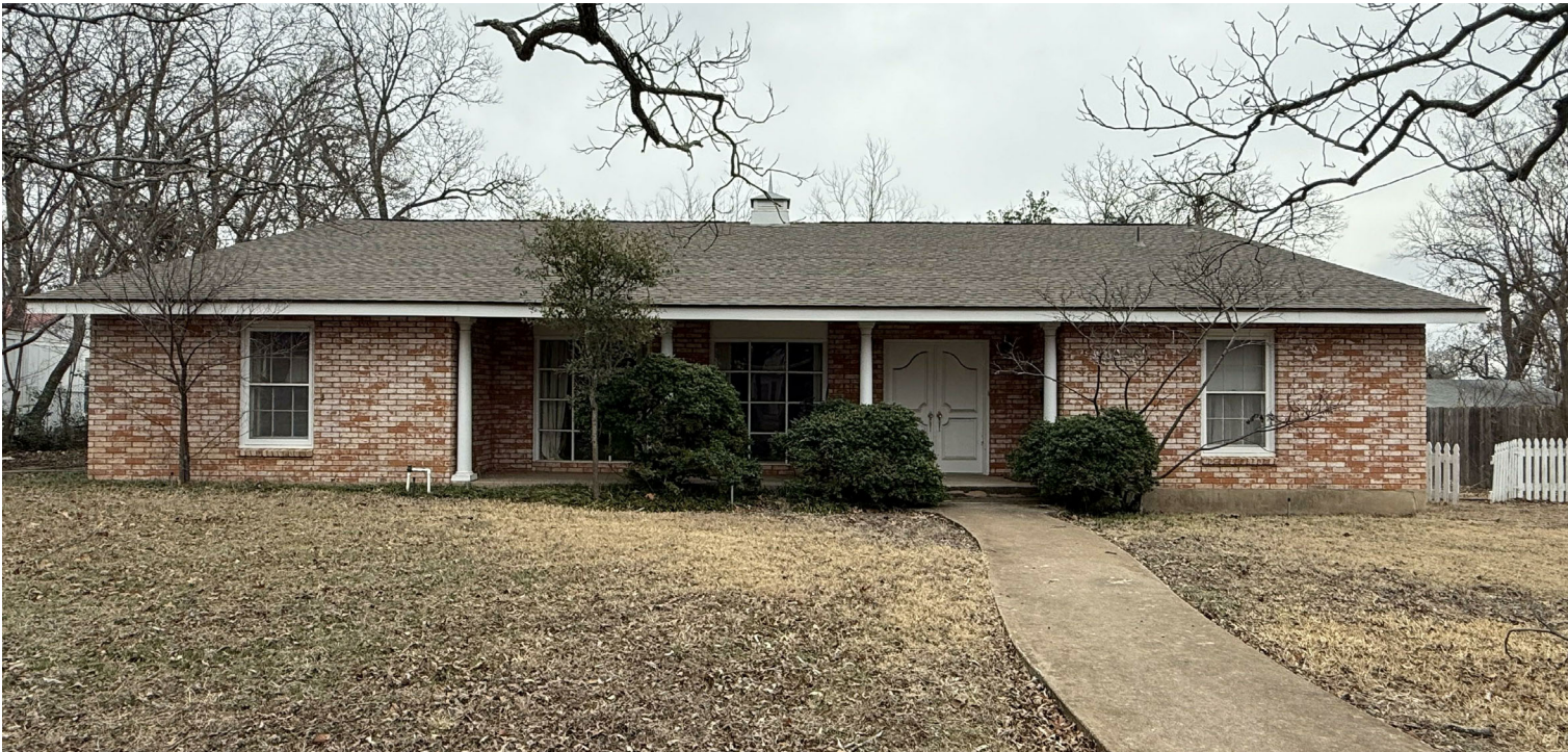
EXISTING RESIDENCE - VIEW FROM SOUTH CROCKETT STREET
