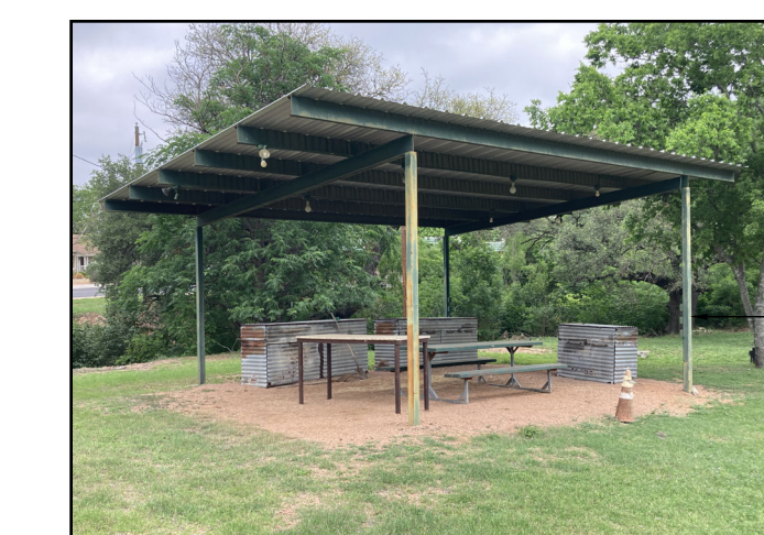
PHOTO #6 - BBQ SHED
