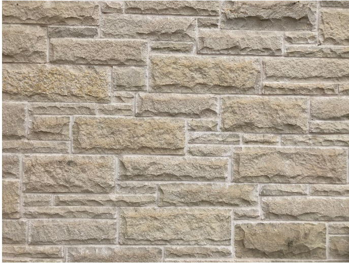
Limestone, split face with saw cut back and edges – photo of existing Bethany Church
