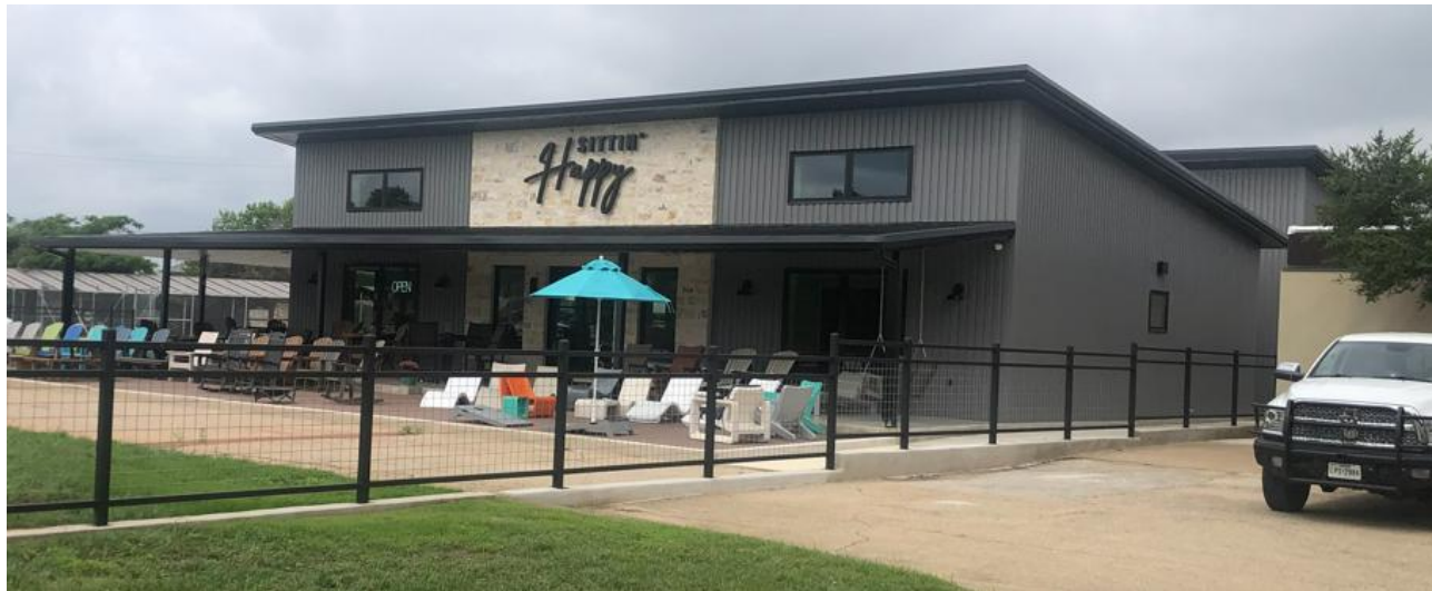
EXISTING CORRIDOR BUILDING WITH SIMILAR COLOR ON HWY. S. 87.
