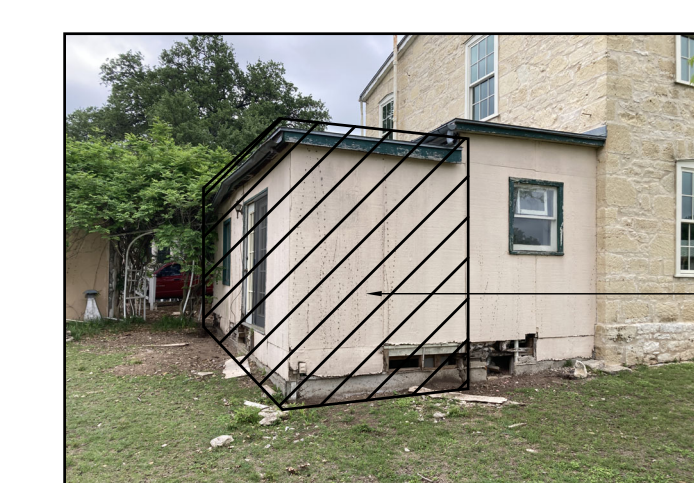
PHOTO #8 - BUILDING ADDITION DEMO BY OWNER
