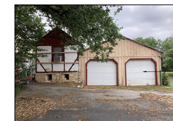
PHOTO #5 - SHED ADDITION
