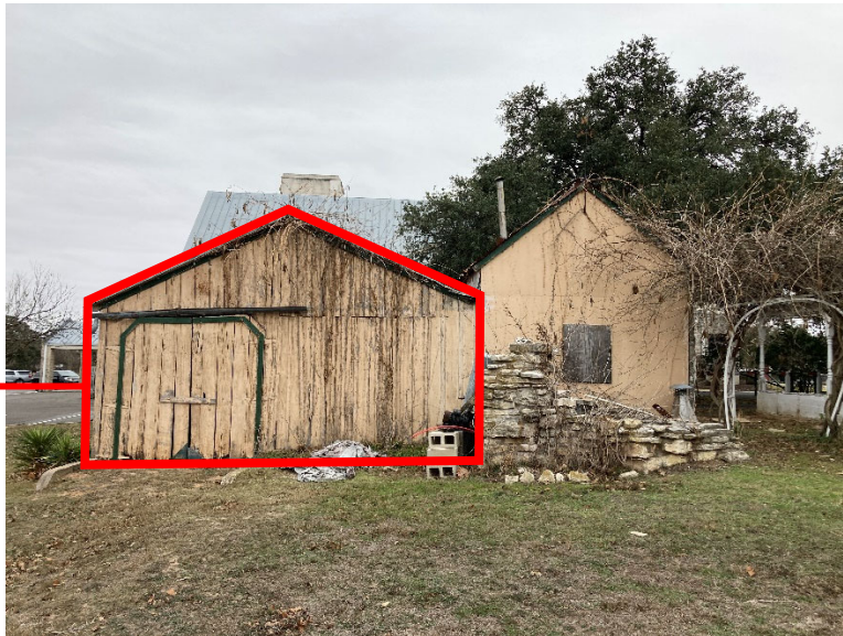
Fachwerk Structure behind the Felix Van Der Stucken Building West Elevation
