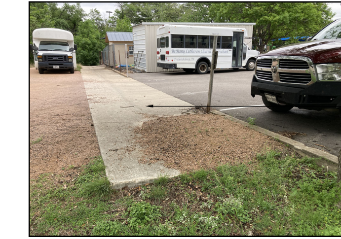
PHOTO #3 - CONCRETE SWALE
