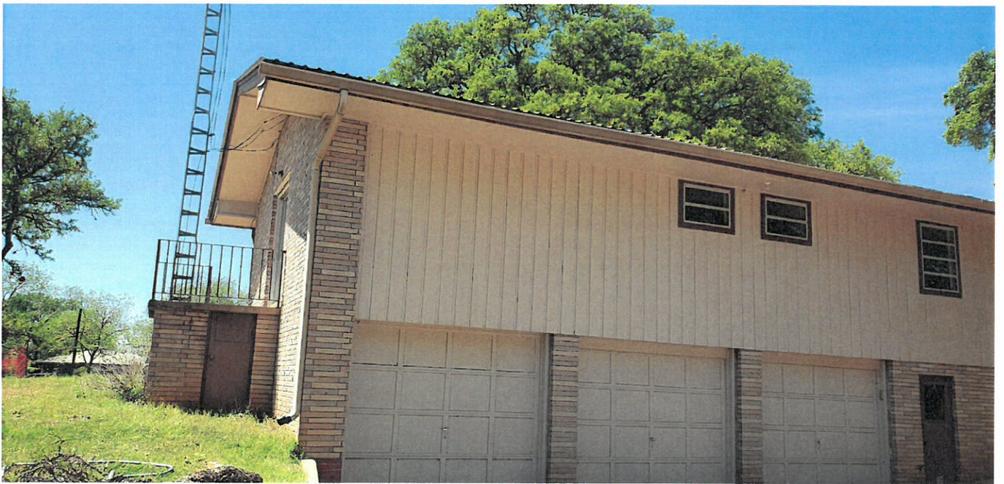
3 bay garage with bedrooms above
