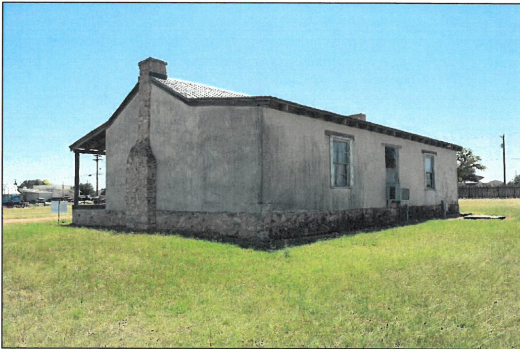
Figure B-14. Building B, Officer's Quarters, facing west.
