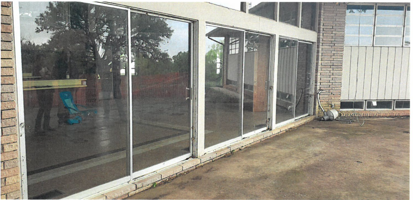
Sliding glass doors from kitchen into courtyard
