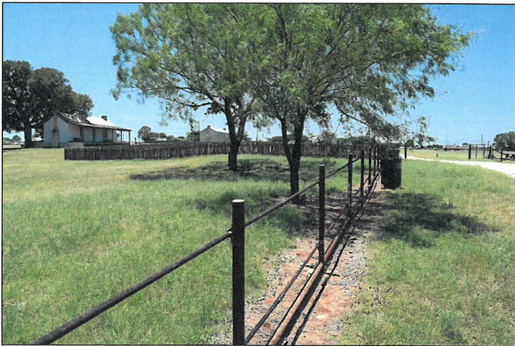
Figure B-6. Partially complete pole fence along north side of fort, facing west.
