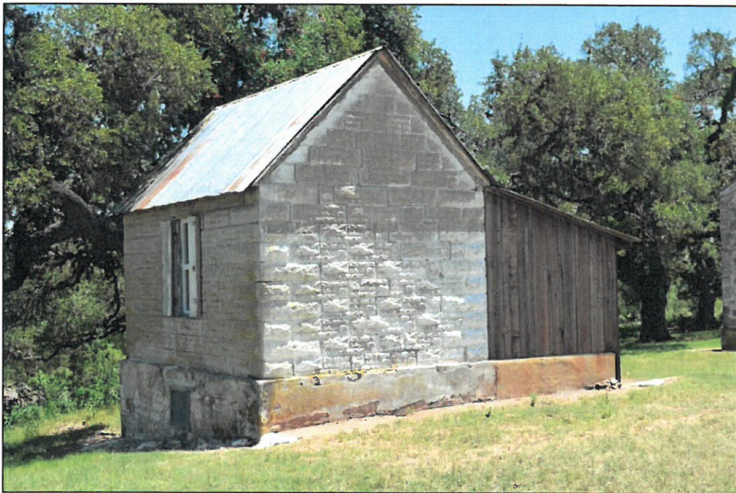
Figure B-34. Wash House (Braeutigam Shed), facing south.
