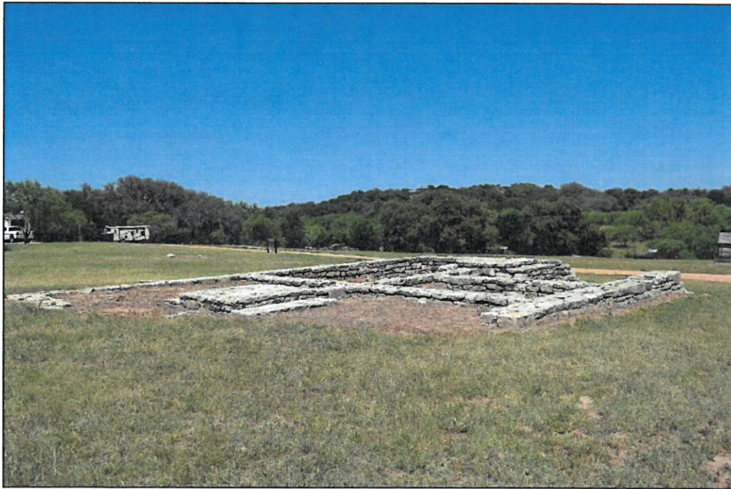
Figure B-22. Building G, Officer's Quarters Foundation, facing northeast.
