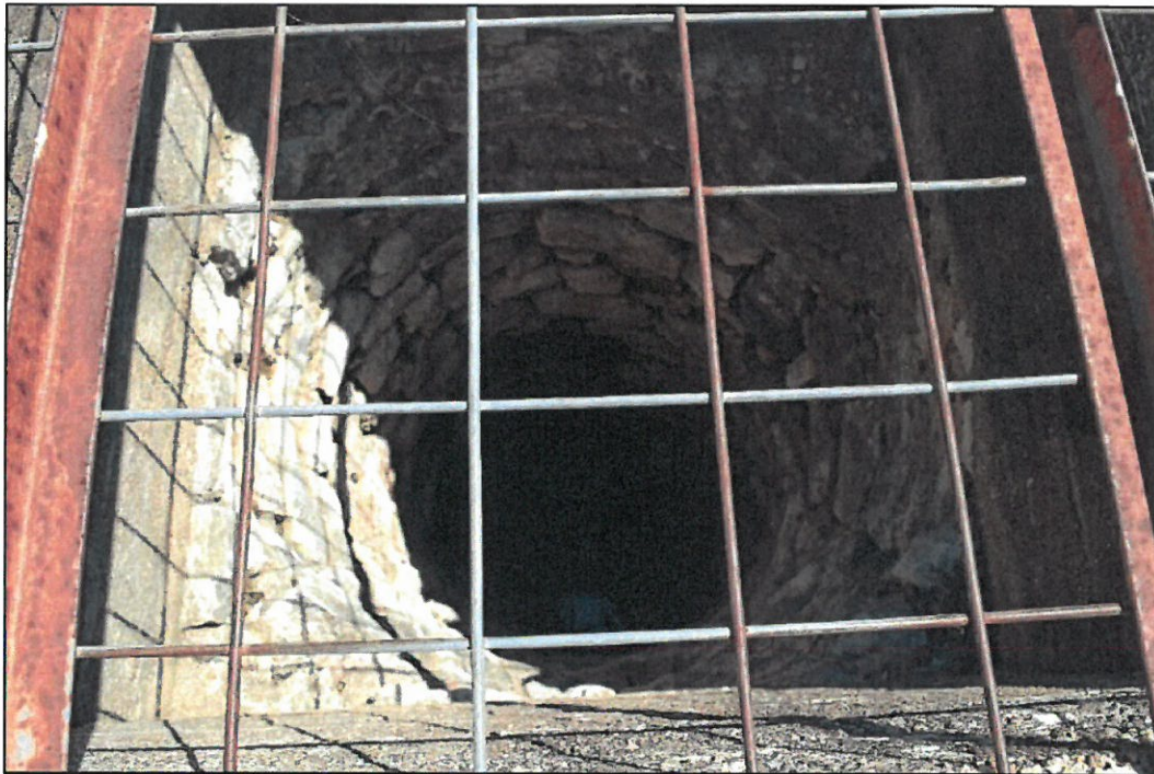
Figure B-37. Interior of Braeutigam Well #1.
