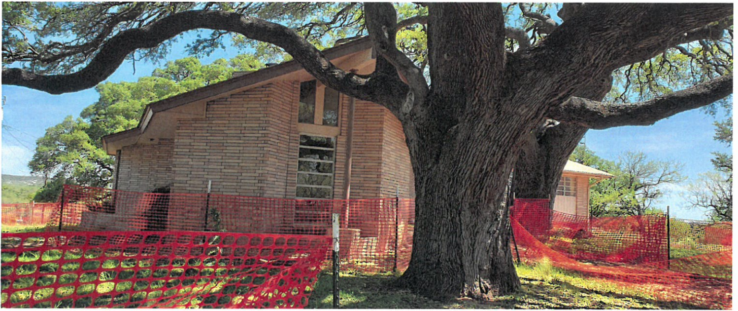
Cantilevered projecting gable
