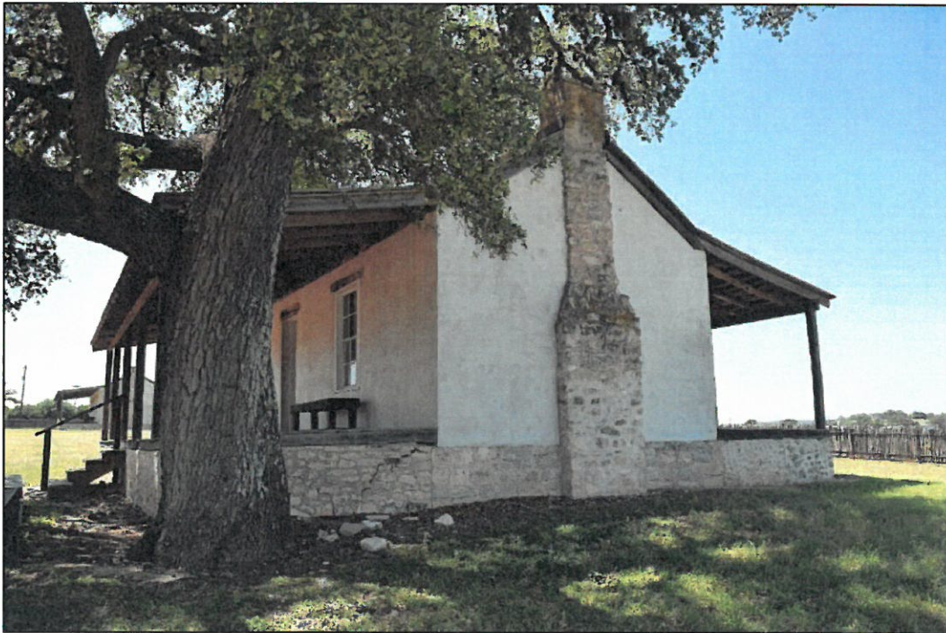
Figure B-18. Building E, Officer's Quarters, facing northwest.
