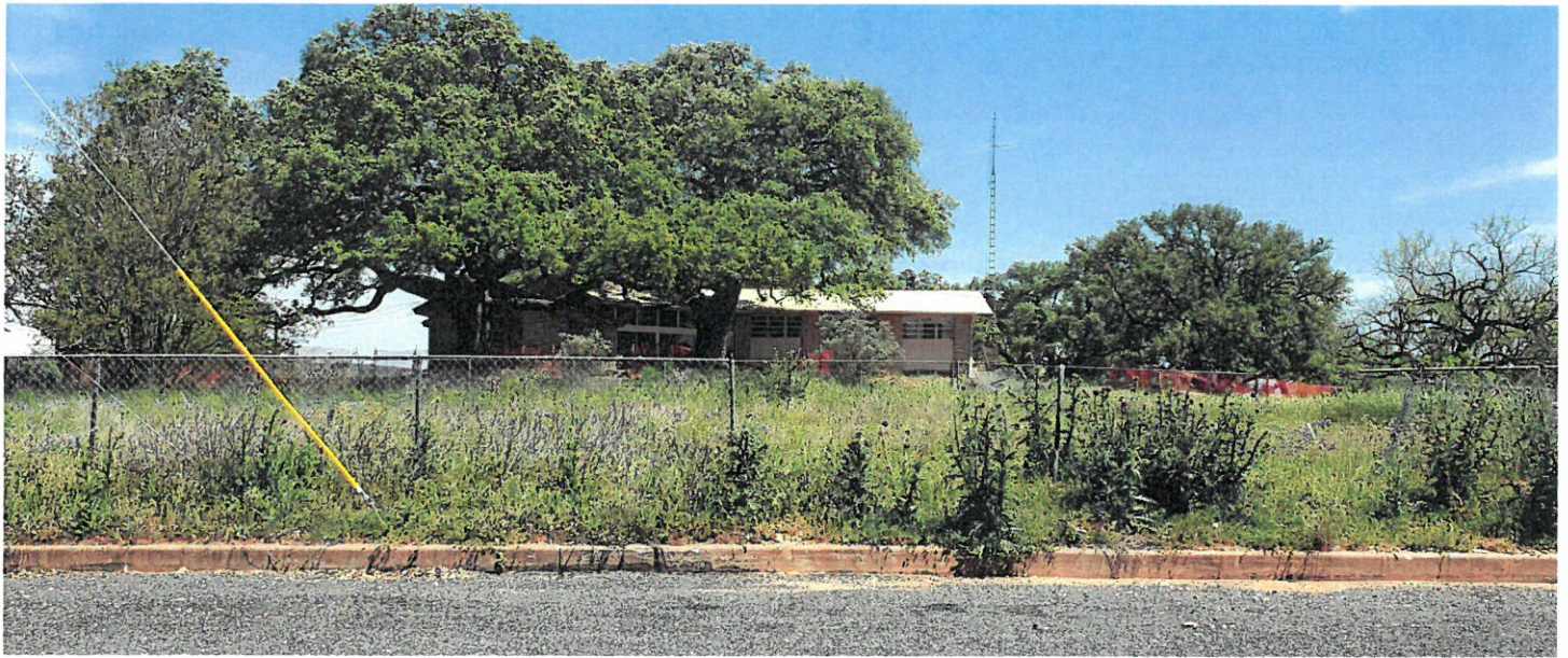
View from E Centre Street looking north
