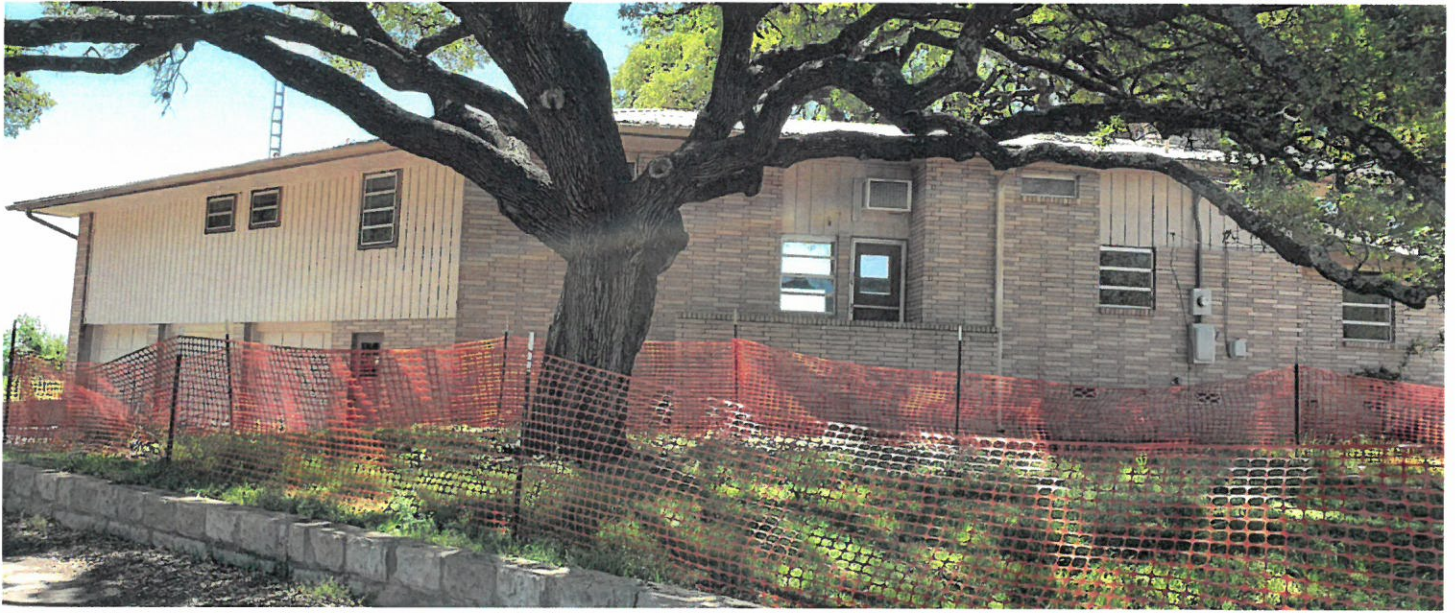
Rear elevation as seen from driveway
