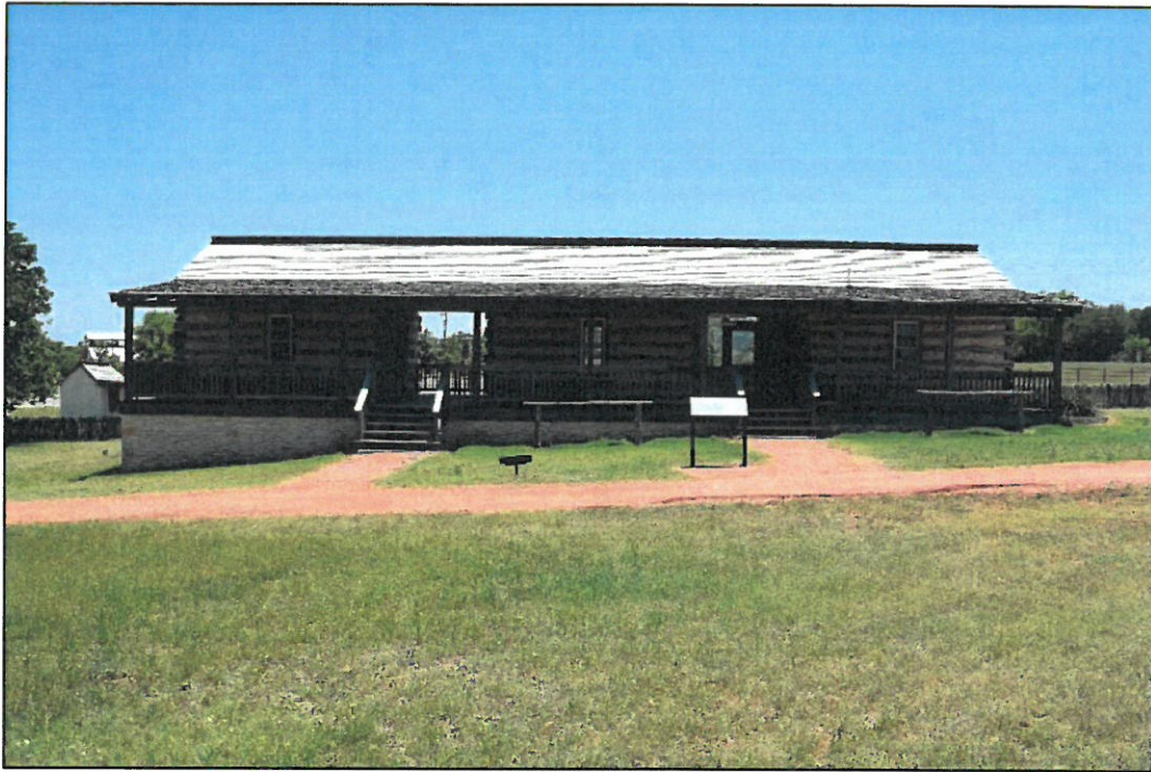
Figure B-39. Building R, the Enlisted Men's Barracks, facing southwest.
