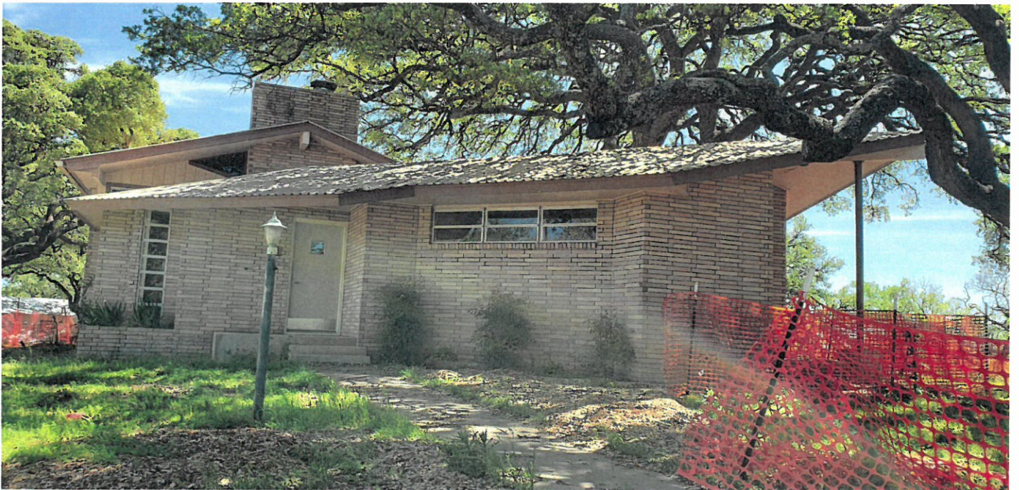
Front door as viewed from N. Elk
