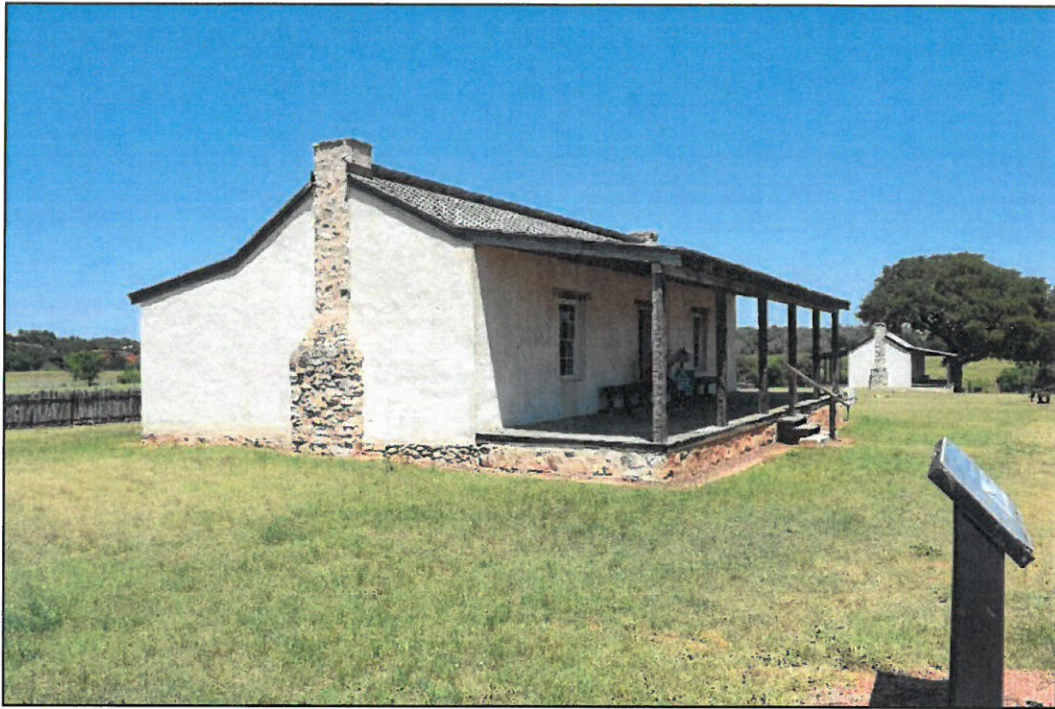
Figure B-13. Building B, Officer's Quarters, facing east.
