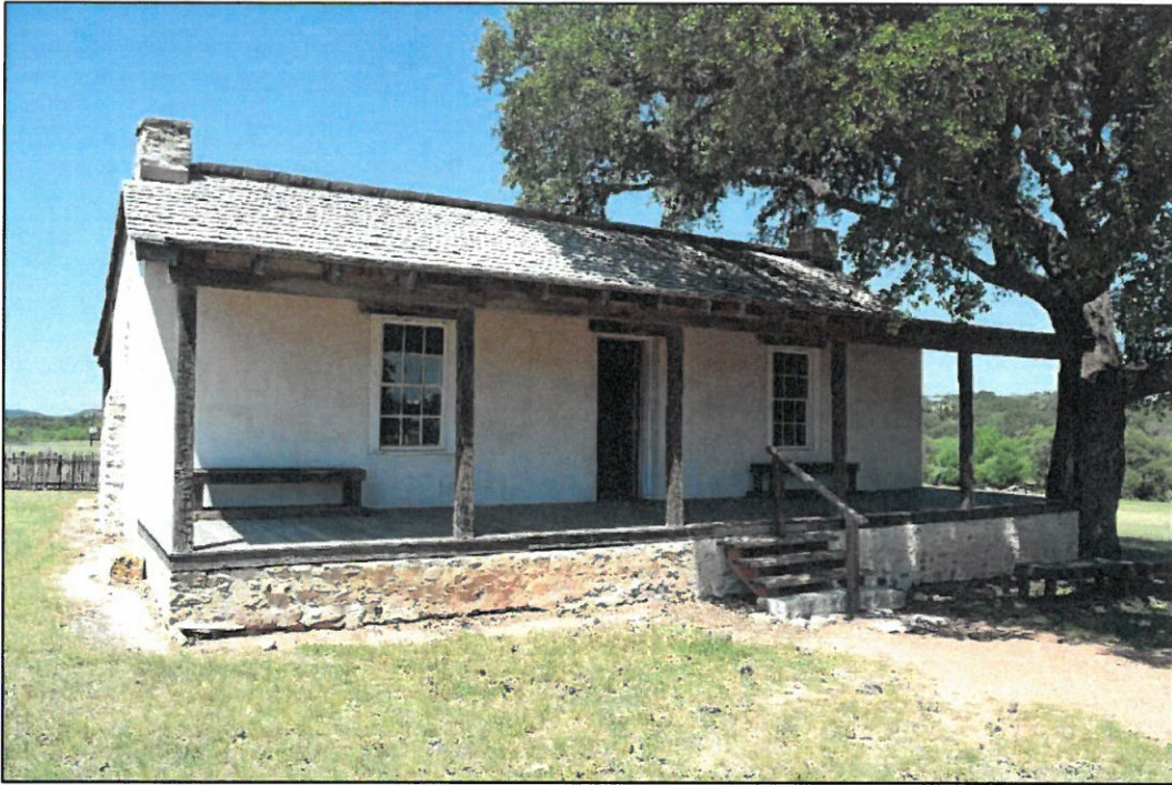
Figure B-17. Building E, Officer's Quarters, facing northeast.
