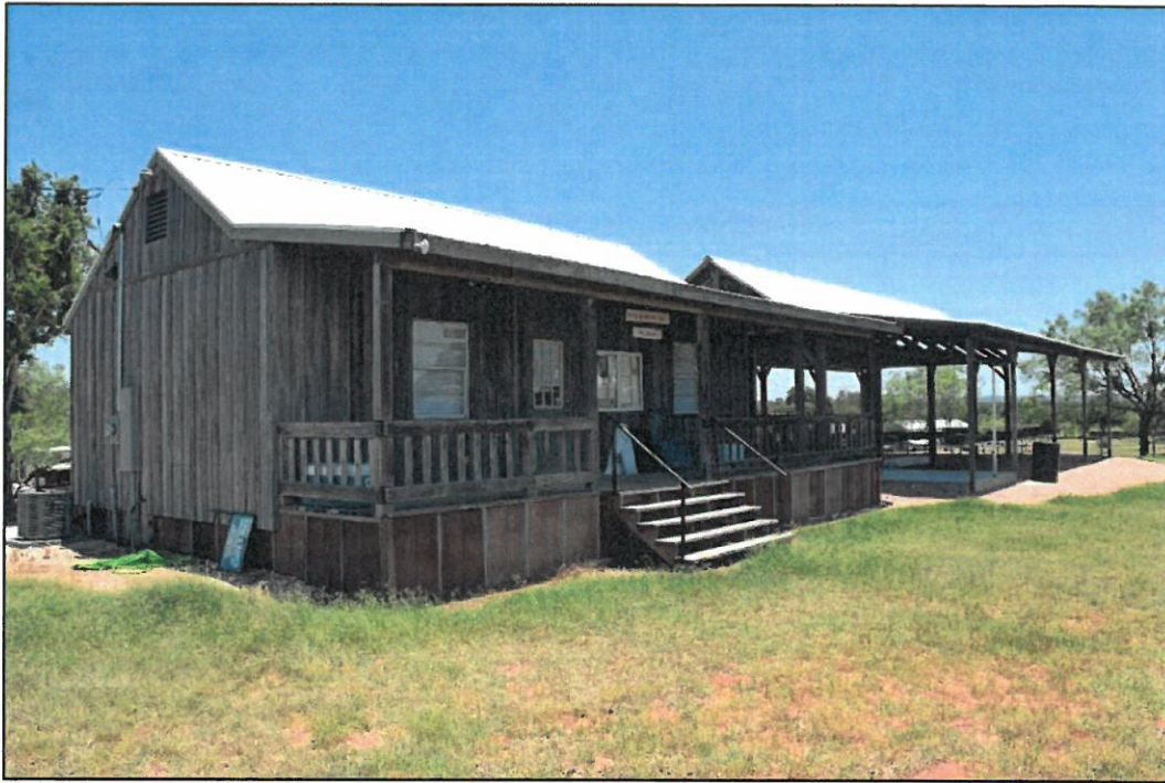
Figure B-47. Friends of Fort Martin Scott Building, facing south.
