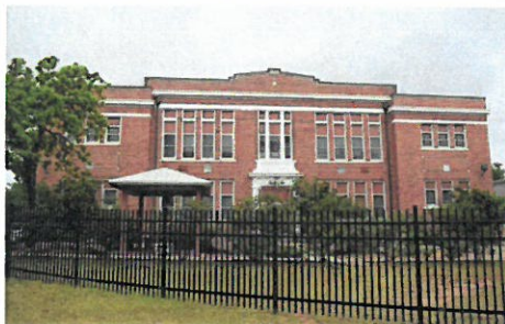
Image 22. 110 W. Travis St. (Survey ID #295A). Former Fredericksburg High School constructed in the Beaux Arts style in 1922 by noted architect H. F. Kuehne. Recommended local landmark and recommended eligible for the NRHP.
