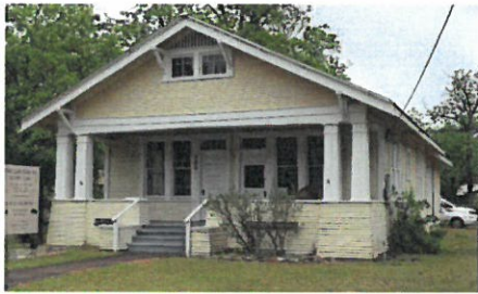
Image 20. 409 N. Milam St. (Survey ID #207). Craftsman style multi-family residence constructed c. 1920. Recommended local landmark.
