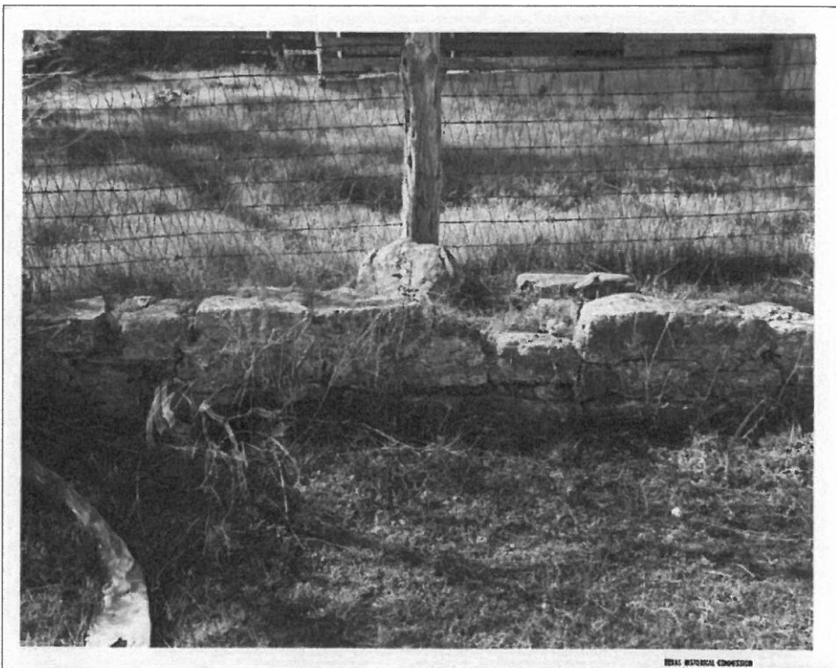
Figure 5. Detail of stone foundations of ruins, specific building and view not noted (NRHP 1979).
