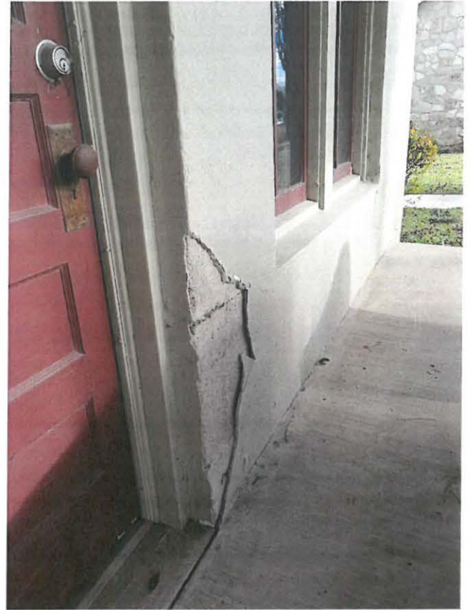
Exterior plaster sluffing due to rising damp, concrete block exposed
