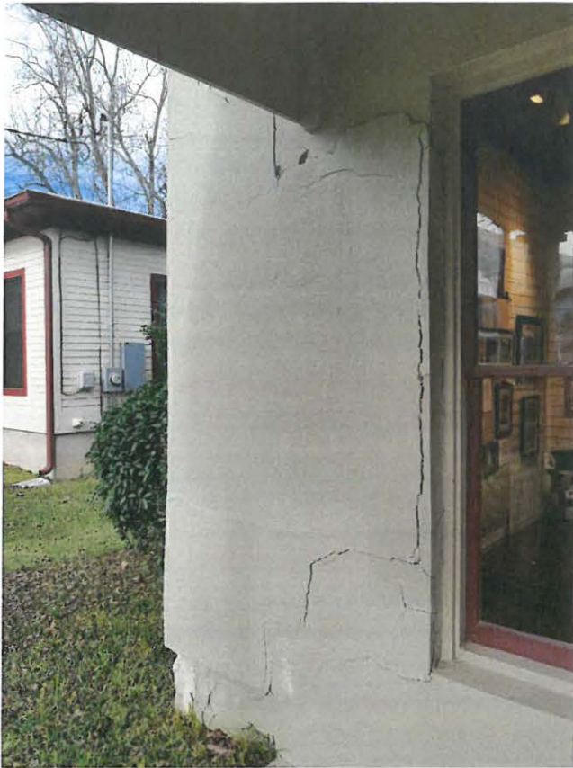
Exterior plaster sluffing due to rising damp, concrete block exposed
