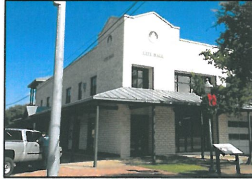
Figure 4: Fredericksburg City Hall
