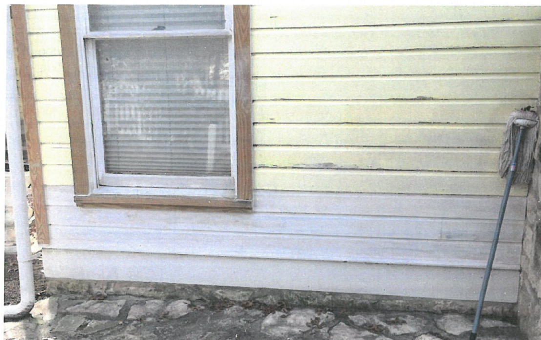
Current siding repair work on later rear addition
