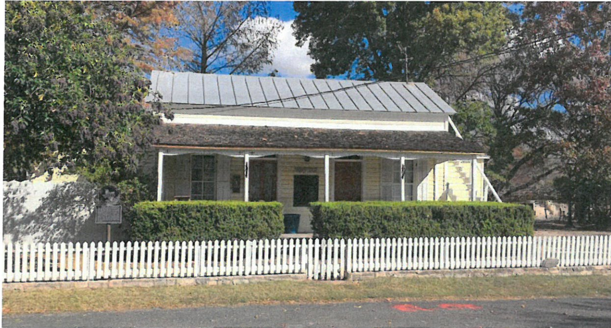
South Elevation facing Schubert Street
