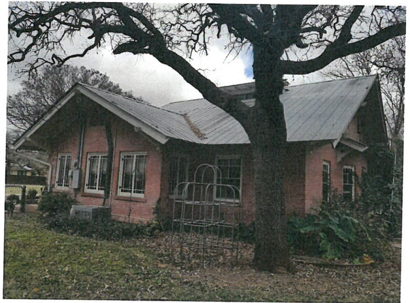
Rear oblique view showing 2nd floor pop up
