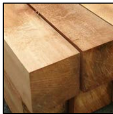
TIMBERS (LOCATION: FRONT PORCH)
