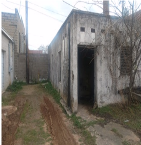
Pictures of original structures of Weidenfeller Building. Approx. 1258 sq. ft. of storage buildings scheduled for demolition and remodel.
