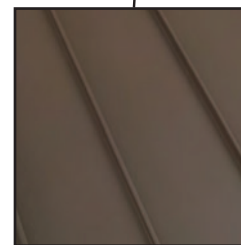
PRE FINISHED BROWN STANDING SEAM METAL ROOF
