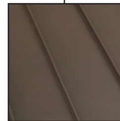
PRE FINISHED BROWN STANDING SEAM METAL ROOF
