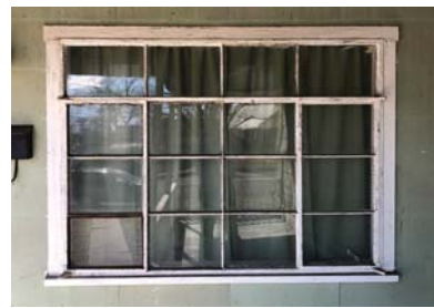
EXISTING STEEL CASEMENT WINDOW
