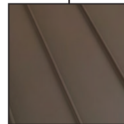
PRE FINISHED BROWN STANDING SEAM METAL ROOF
