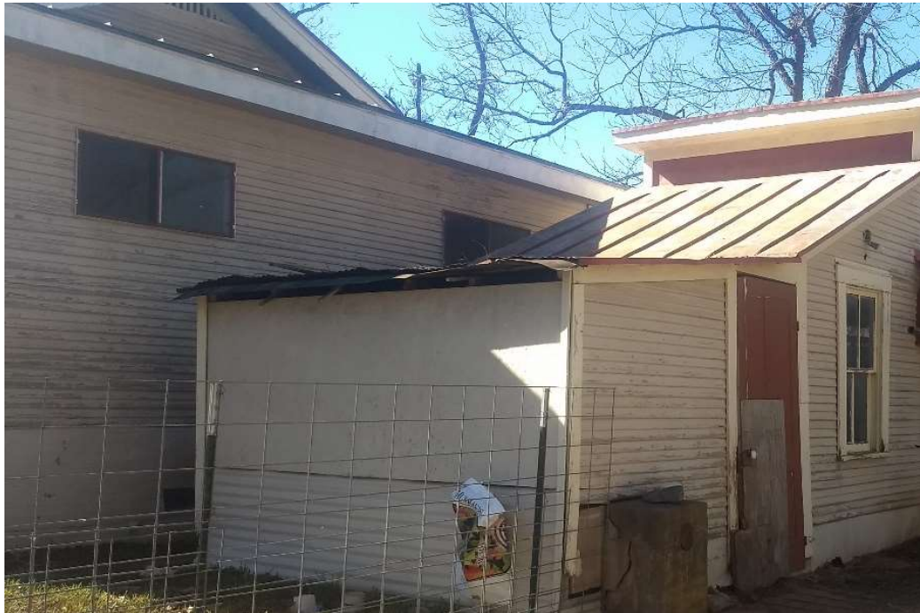
Photo 5 – rear of house – view obscured by sheds built very close to house
