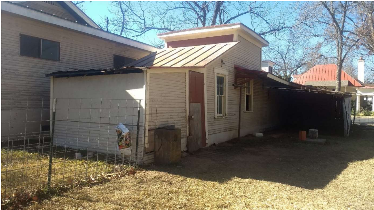
Photo 8 – Sheds tacked onto Tank House and Garage
