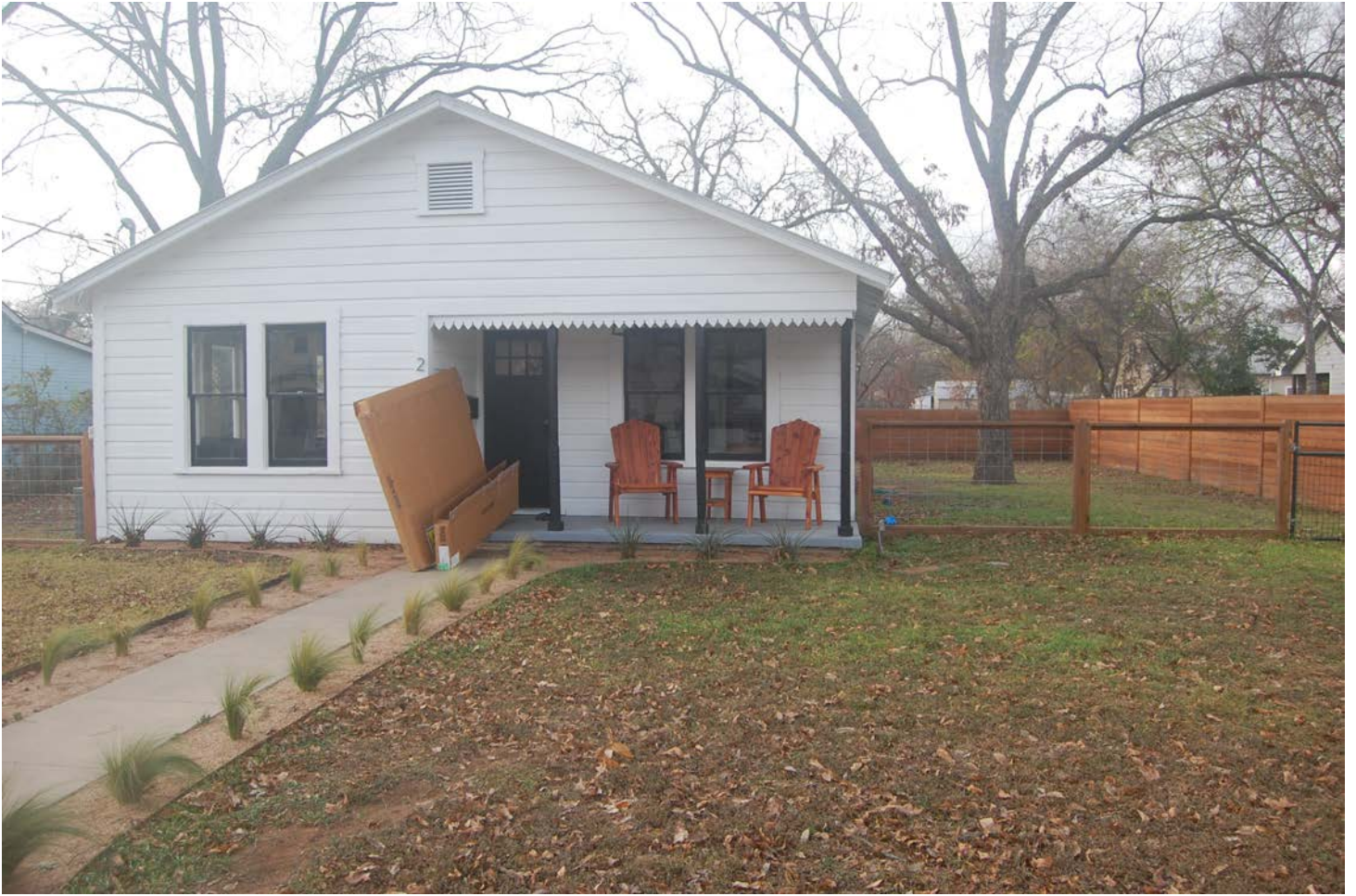
4 S. Bowie Street view north side of house, location of new addition (behind tree)
