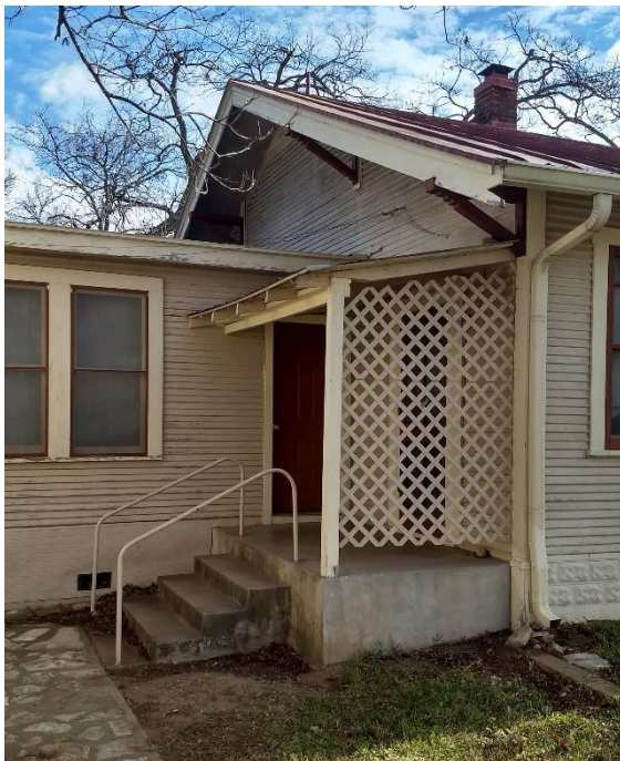
Photo 6 & 7 – Back Porch – next to room addition
