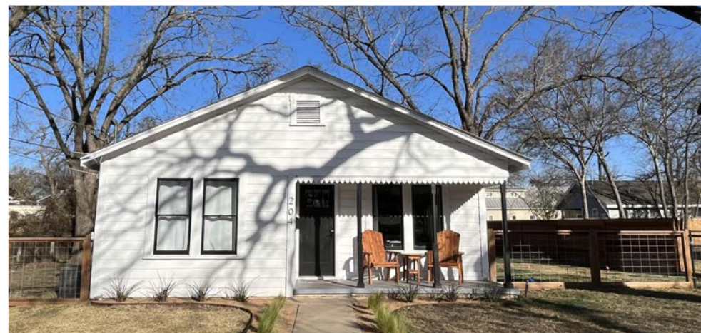
EXISTING BUILDING FRONT ELEVATION
