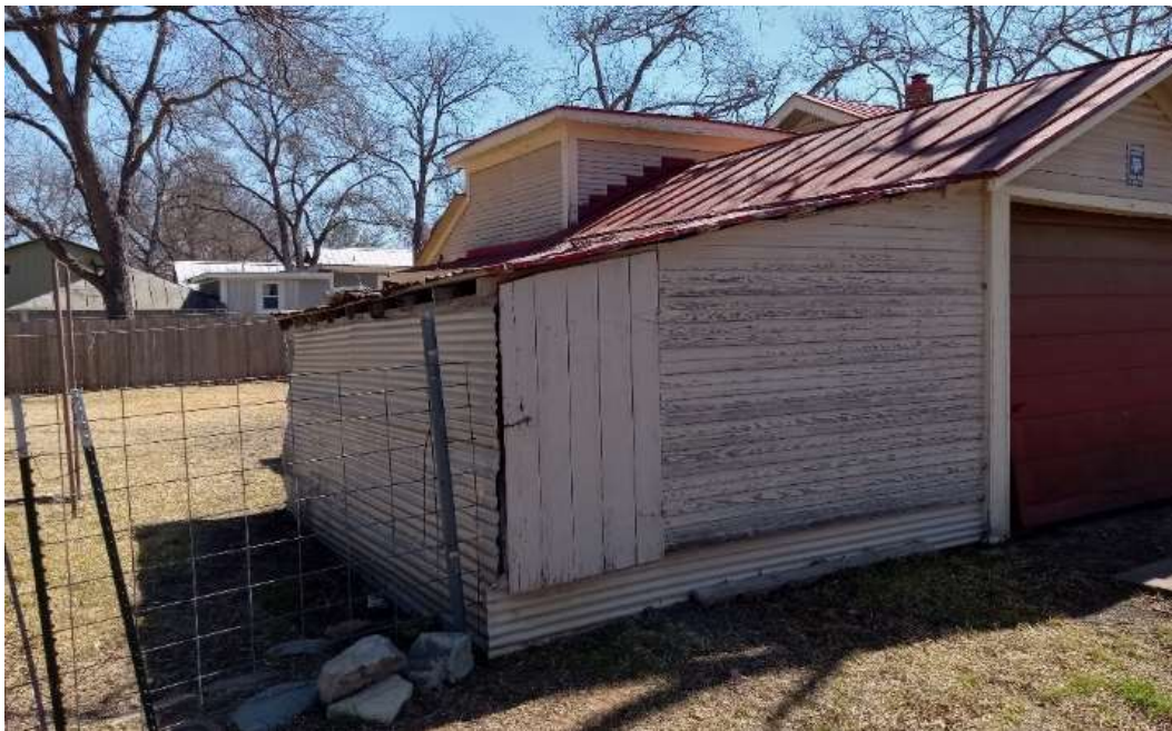
Photo 12 – Street view of equipment shed attached to Original Garage.
