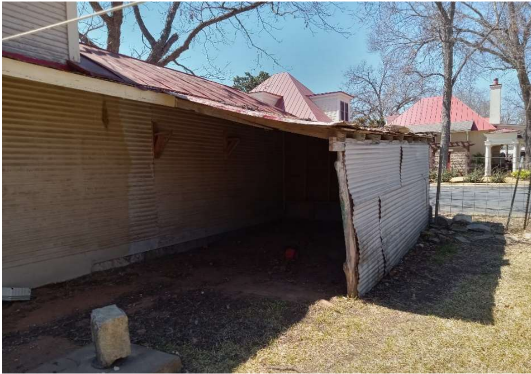
Photo 11 – Shed that appears to be a carport but is not. May have housed lawn equip.
