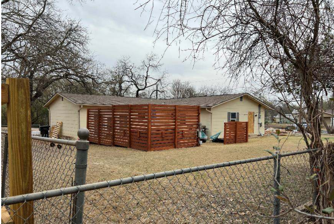
304 N Bowie – South West Corner of Property
