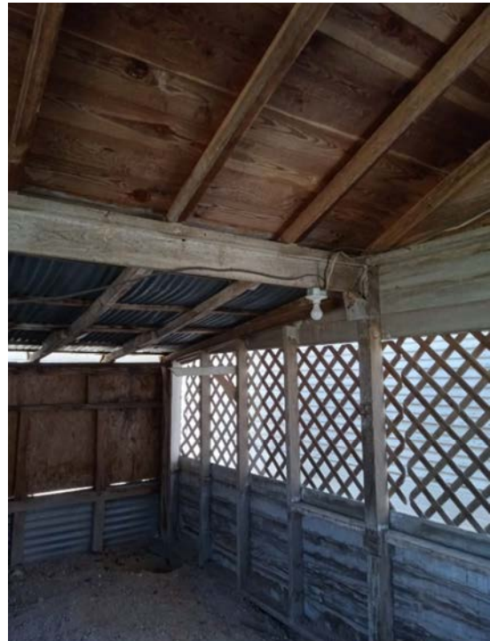
Photo 10 – interior of sheds
