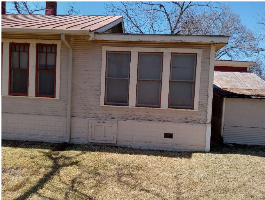
Photo 4 – detail of room addition
