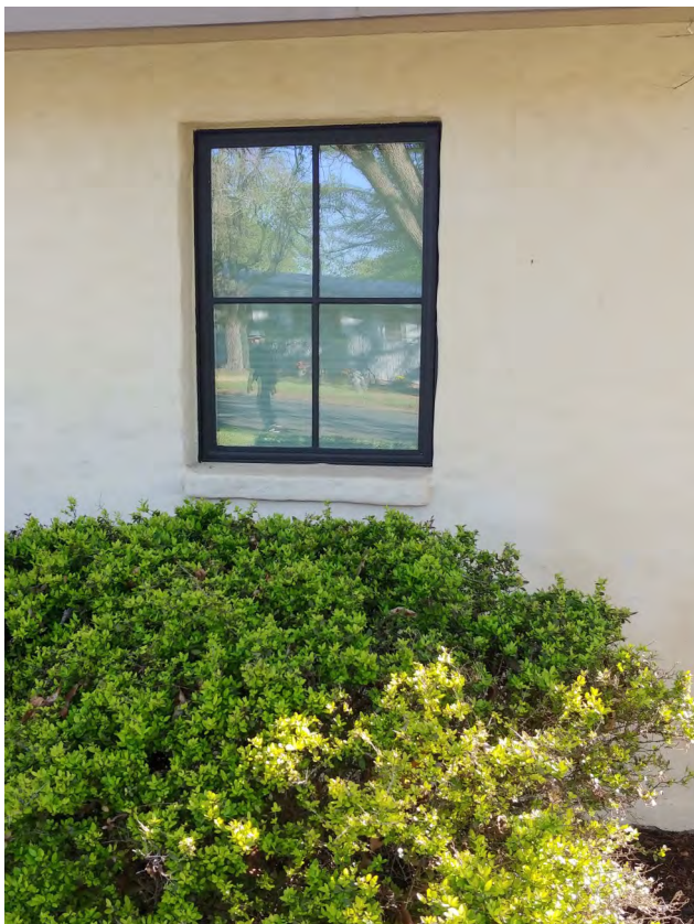
Two aluminum windows to be replaced to match original windows
